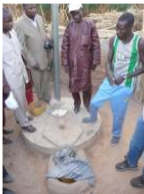
Abass show his composting latrine with urine diversion.
