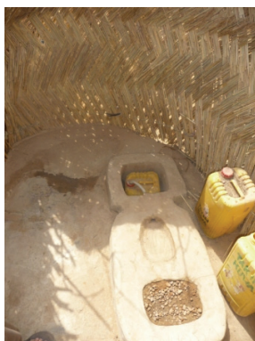
An improved urinal at the house of one of the masons
