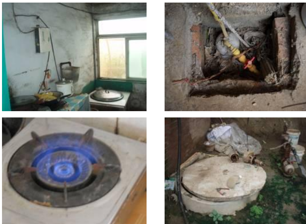
Figure 17: Biogas system components
