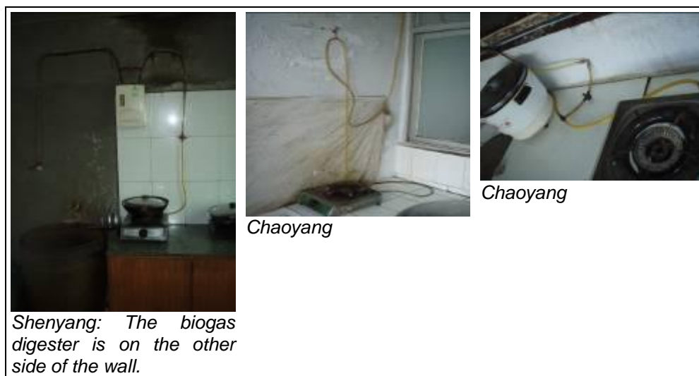
Figure 19: Inside gas pipelines
