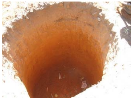
The pit is dug 1.7m wide and 2m deep. Walls are straight and bottom flat
