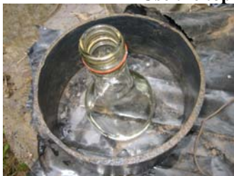
Encase the bottle top on concrete and allow to cure
