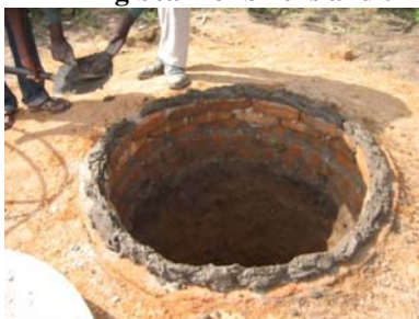
Ring beam of bricks and three courses of corbelled brickwork
