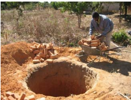
The pit is dug 1.7m wide and 2m deep. Walls are straight and bottom flat
