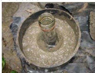
Encase the bottle top on concrete and allow to cure
