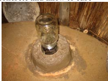
Mount the mounted bottle top over the vent hole and cover with a jam jar
