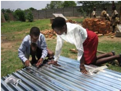
The nails should be driven through the tin sheet and made tight in the wood.
