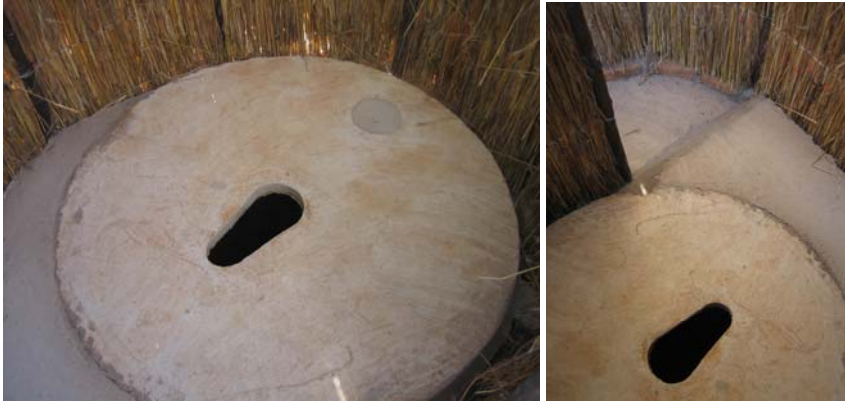
The concrete floor is extended in front of the slab and also within the spiral entrance. The vent hole has been temporarily plugged.
