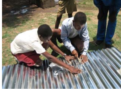
Three sheets are used each 1.5m long. These are cut from 3m sheets. The three sheets are fastened to the wooden frame with small nails with large heads. Each sheet overlaps the one next to it.
