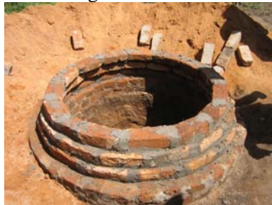
Ring beam of bricks and three courses of corbelled brickwork
