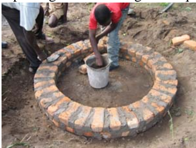
Ring beam of bricks and three courses of corbelled brickwork
