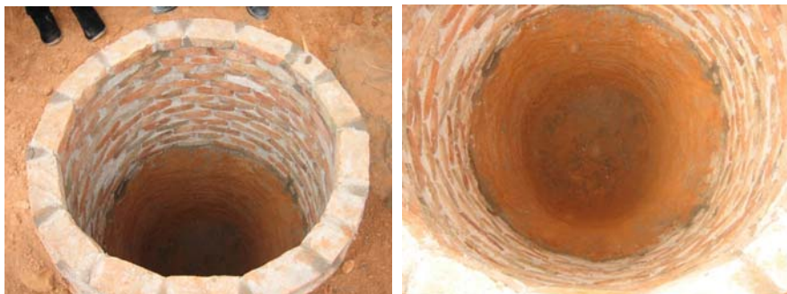
A partially lined pit used in firmer soils.
