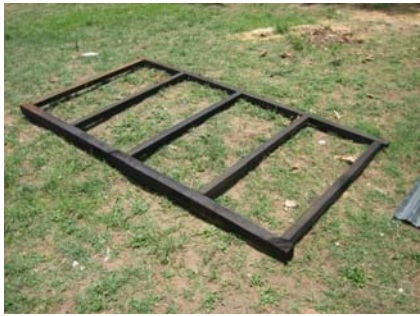
The untreated and treated wooden frame which is nailed together
