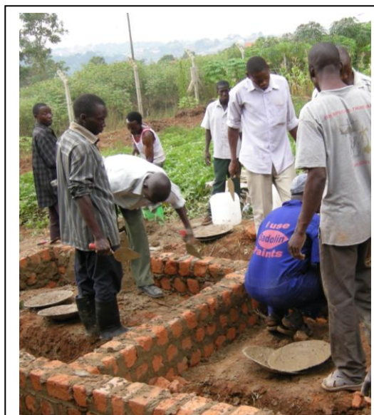
Training of masons in UDDT construction, Mukono, Uganda
