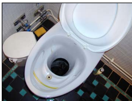
Figure 2: Dry urine-diversion toilet (Source: Wostman Ecology)
