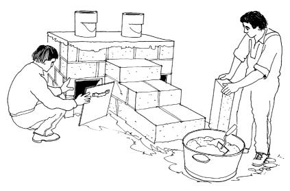
Figure 3.3 A Last toilet under construction. On top of each vault is a seat riser with a urine collector. The seat riser not in use is usually covered with a plastic bag.
