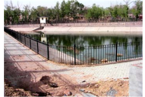
On-site storage pond for treated greywater that will be reused
