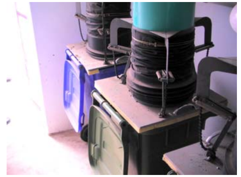
Faeces collection bins
