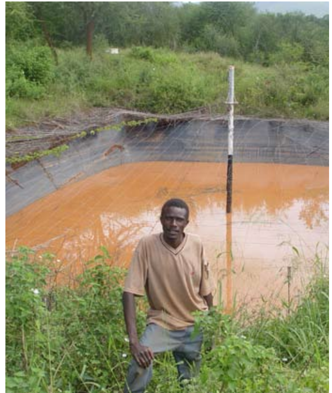
Water harvesting dam for supplemental irrigation. Photo: A Odior, ICRAF
