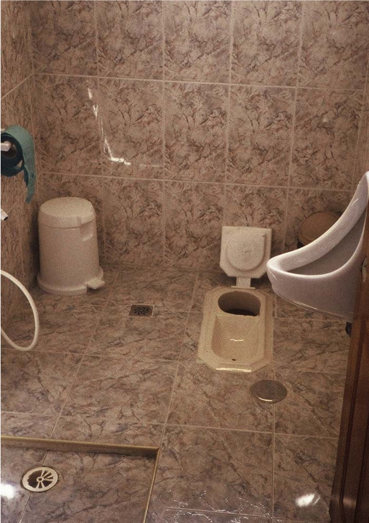
Fig 2: A typical toilet room in the PHG project . The lid is open and the drop hole for faeces is visible. To the left of the squatting pan is a drain for anal cleaning water. The bucket further to the left is for soiled toilet paper.
