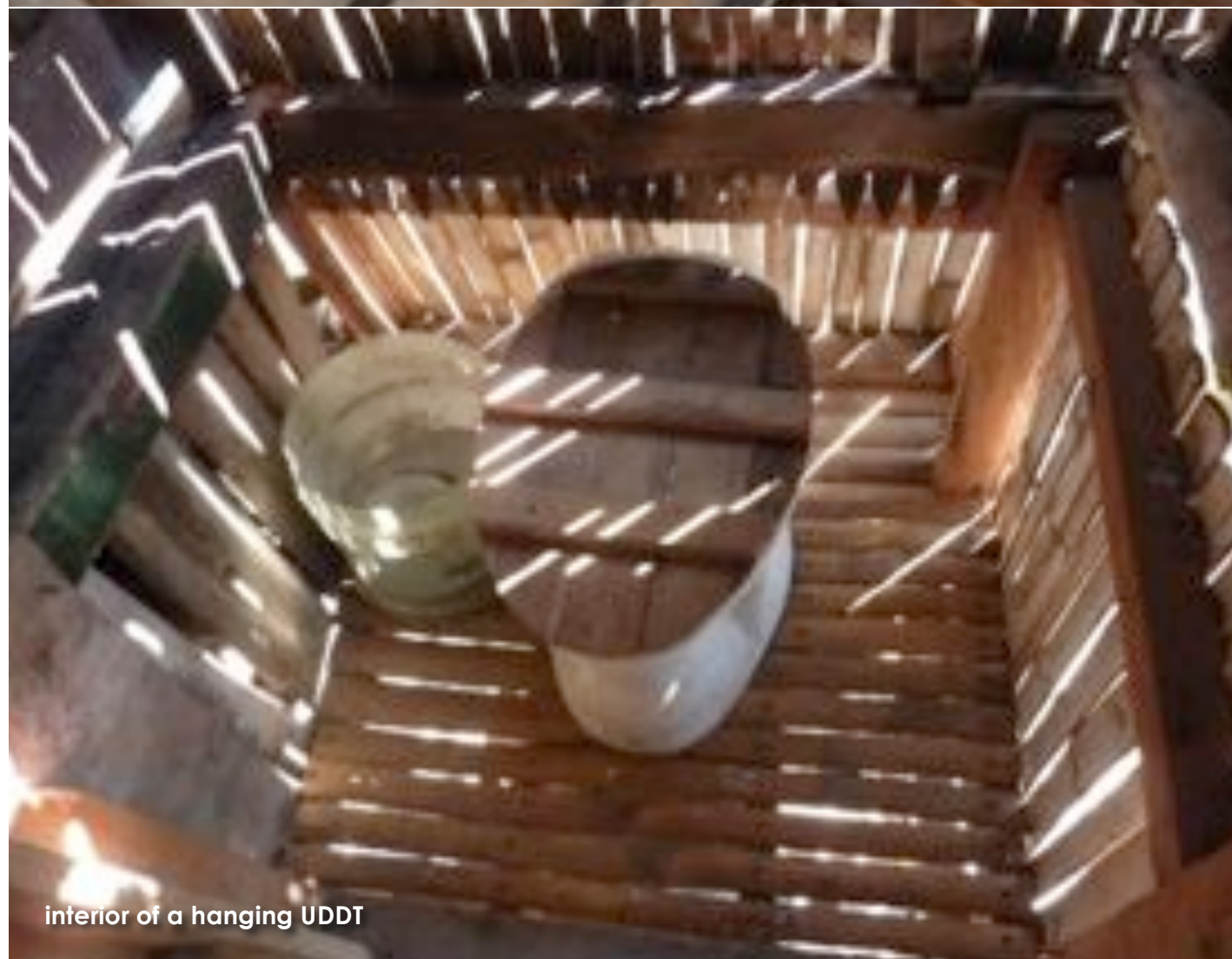
interior of a hanging UDDT with user instructions on the door
