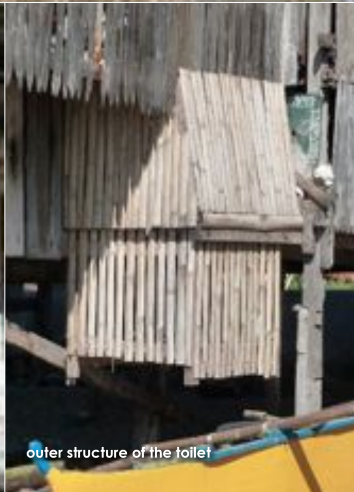
hanging UDDT in a house along the coast in Initao, Misamis Oriental
