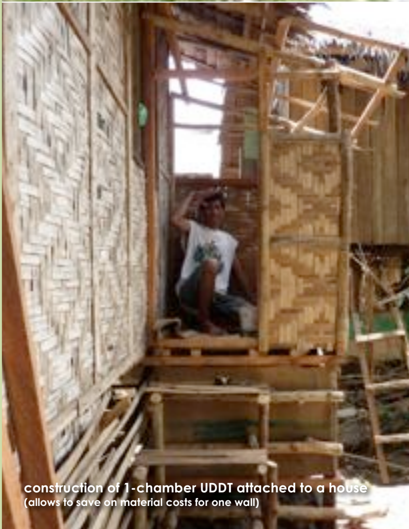
low-cost 1-chamber UDDT (with amakan walls and nipa roof)
