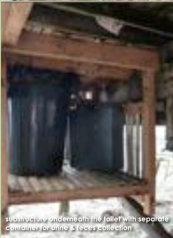
hanging UDDT in a house along the coast in Initao, Misamis Oriental
