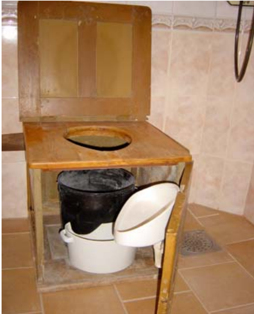
Figure 2. Urine-diverting toilet from 1863 with urine funnel and collector (broken) in porcelain, and faecal container of metal sheet. (Photo Drangert 2001)
