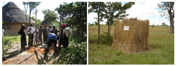
This house structure is used to make the place private. There are many ways of making the house structure. It is best to make a roof to fit over the structure for shade and to keep the rain out.
