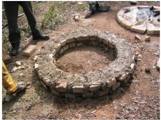
Then dig out the pit inside the ring beam down to 1 metre or even 1.5 metres below ground level. Some of the soil which comes out of the pit is placed around the ring beam and rammed hard in place. This will help to make the ring beam strong in its place.
