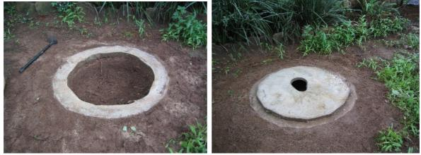
Dig down hole within the ring beam to at least 1 metre below surface. Place soil around ring beam and ram in place hard. Add leaves to pit base. Lay anthill mortar or weak cement on ring beam and place slab on top. Bed in and level the slab. The structure can now be built around the slab.
