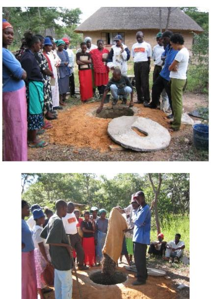
First put a big sack full of dry leaves in the pit The leaves will help the contents of the pit to compost. Then lay the slab over the ring beam
