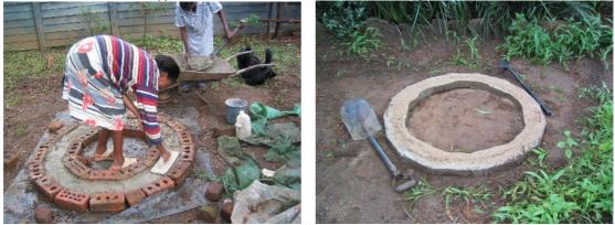
Add remainder of concrete mix, level off and ram flat with wooden float. Cover with plastic sheet and leave to cure for 10 days. Keep wet at all times. Then move to location on level ground.
