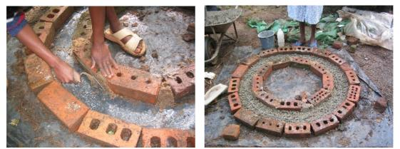
Fill in spaces between inner circle of brick mould with wet sand. Make the 6:1 mix of clean river sand and fresh cement. Add half the mix, level off and then add the circle of 3 – 4mm wire
