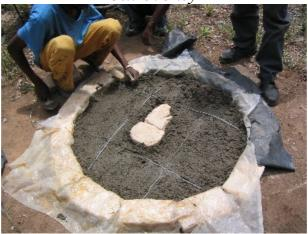
Add 4 reinforcing wires each 3 to 4mm in diameter and 90cm long in a square shape around the squat hole. Then add the rest of the concrete mixture. Spread out evenly. Also ram down hard with a wooden float. Smooth off with a steel trowel. Add two thick wire handles on either side for lifting.
