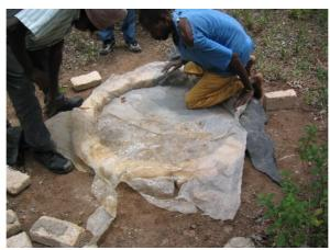
The squat hole is made by placing a shaped plastic bucket or shaped bricks in the slab mould.
