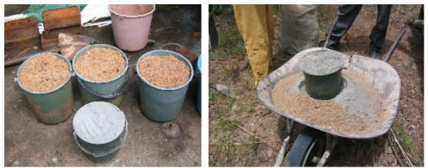
The sand and cement must be very well mixed. After mixing the dry sand and cement add water (about 2 - 3 litres) to make a stiff mix. Mix thoroughly again. Add half the mix to the slab mould and spread out evenly
