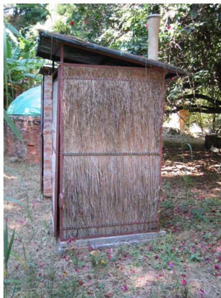
Front and side views of the superstructure frame covered with grass
