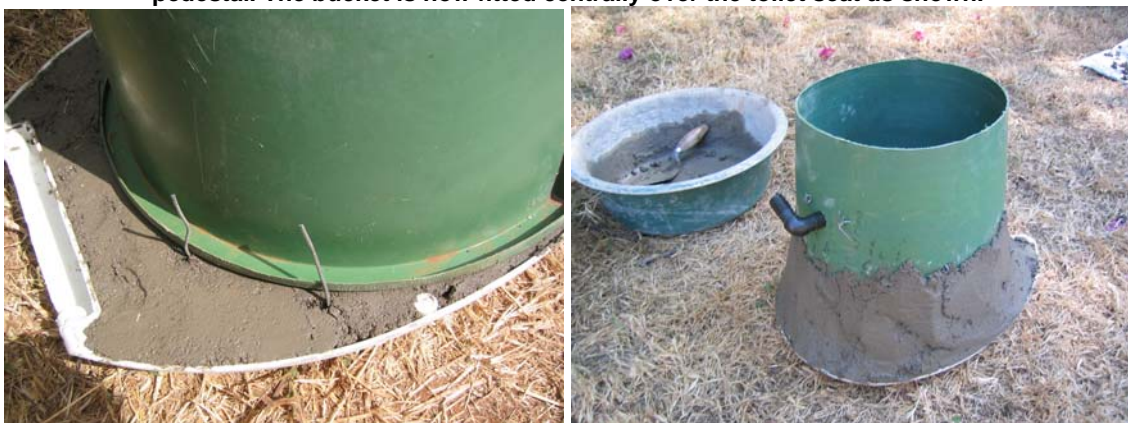
8 pieces of bent wire are now introduced into the cement supporting the seat. This is allowed to cure overnight. Next a further mix of 3:1 sand and cement is made and plastered half way up the walls of the bucket. This is left overnight again to cure.
