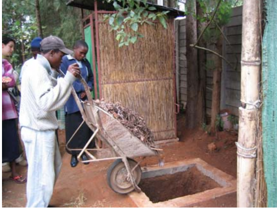
Adding leaves to Fossa alterna pits. On left at Woodhall road, on right at Epworth.
