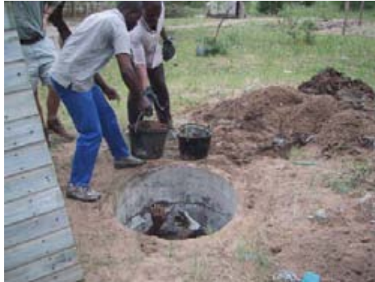
Some work on recycling the existing pit contents of VIP toilets is also being carried out in Maputaland. On the left a previously full pit toilet, to which soil and leaves were added from the top is being dug out three years later. Previously it would have been impossible to dig out by hand. In Maputaland and elsewhere in South Africa, large numbers of VIP toilets were built years ago and many are now full.
