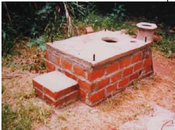
The vault access slab and the toilet slab have now been fitted. The superstructure must now be made.
