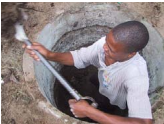
Some work on recycling the existing pit contents of VIP toilets is also being carried out in Maputaland. On the left a previously full pit toilet, to which soil and leaves were added from the top is being dug out three years later. Previously it would have been impossible to dig out by hand. In Maputaland and elsewhere in South Africa, large numbers of VIP toilets were built years ago and many are now full.
