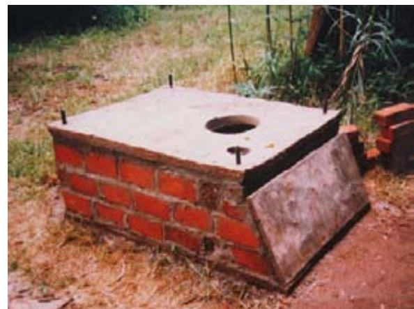
The vault access slab and the toilet slab have now been fitted. The superstructure must now be made.
