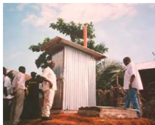
On the left adding semi-composted "makuti," the leaf of the palm tree, to the base of a Fossa alterna to promote composting. On the right a finished Fossa alterna at Bengala Village. Both pits, dug down to 1.5m are fully lined with coral limestone blocks in loose soil. The second pit has been left empty and covered with a tin lid. The addition of soil, wood ash and leaves to excreta promotes composting in the pits. It is this promotion of the composting process which makes the Fossa alterna concept possible.
