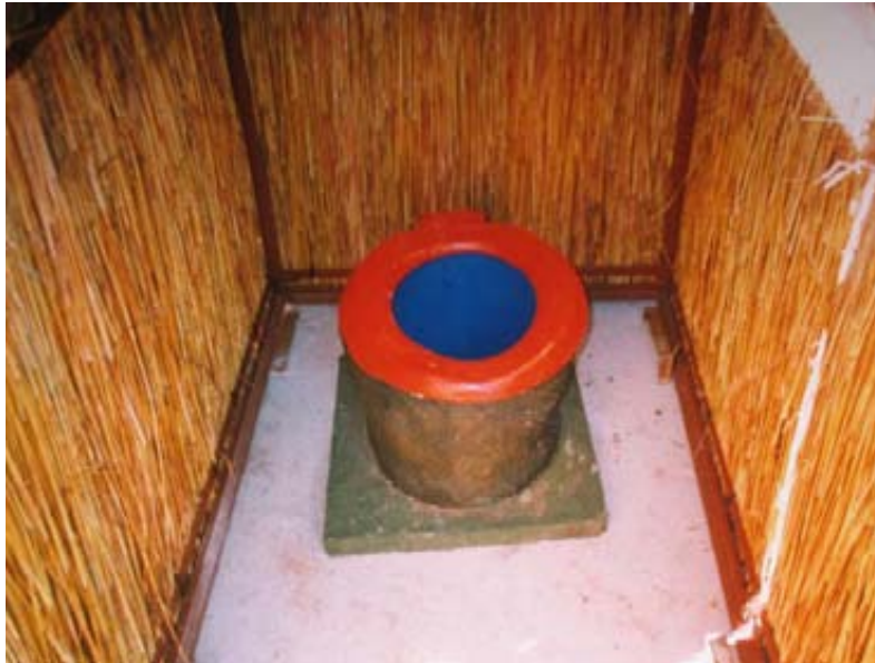
Home made pedestal placed on the slab. The pedestal is smart, cheap and durable.
