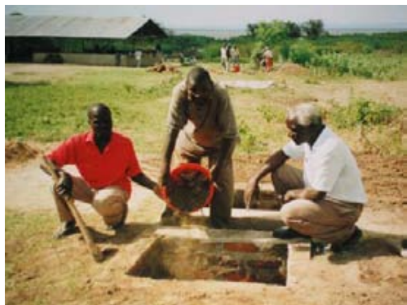
On the left two brick ring beams have been built for a Fossa alterna in Lichinga, Niassa Province Mozambique. On the right two brick ring beams have been built in Kusa, near Kisumu, Kenya. The ring beams are permanently sited and are best bonded with strong cement mortar.
