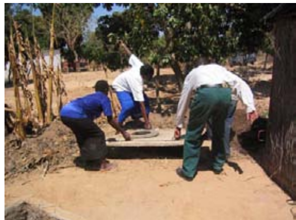
The concrete slab is now removed using the four handles and this is immediately placed over the now empty pit nearby. The slab is levelled and best laid on a bed of weak cement mortar laid over the pit lining brickwork.
