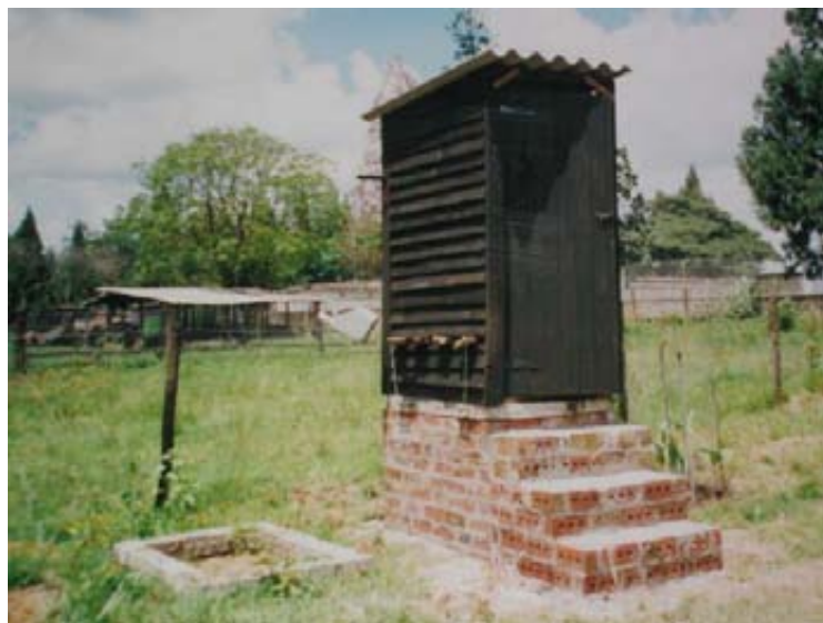
Vault above ground and pit below the ground – used alternately.
