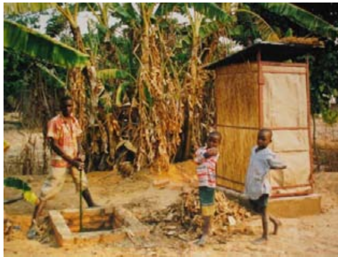
Fossa alterna in Epworth near Harare. It has two shallow pits, a single concrete slab and single superstructure, made with a light steel frame covered with grass. The Fossa alterna was initially designed for per-urban use on medium sized plots, but can be used on smaller plots and also in the rural areas.
