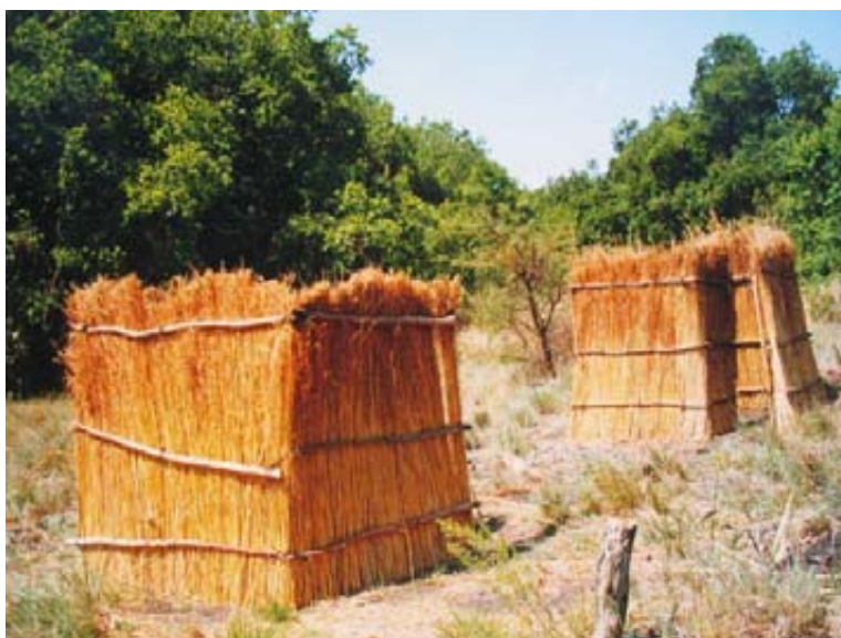
The Arborloo is the simplest ecological toilet. Photo at Eco-Ed Trust.
