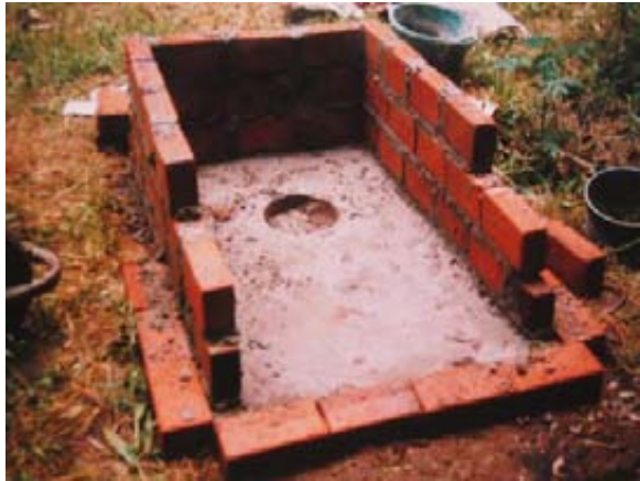
Stages in making the vault. The brickwork
