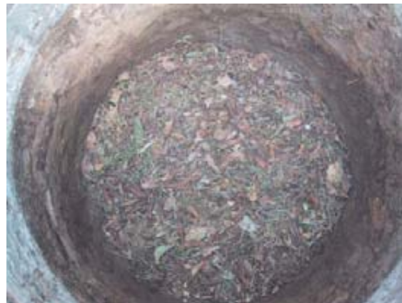
Adding semi composted palm leaves to the base of a Fossa alterna pit in Mombasa, Kenya (left). Two sacks full of leaves at the base of a concrete lined pit in Maputaland, South Africa.
