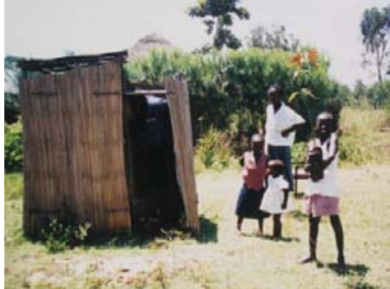
Left, simple portable structure made from poles and grass in Mozambique. This one has no door but has a roof, which has just been removed. The various sections are in panels and can be taken apart. Photo taken in Niassa Province. Thanks to Ned Breslin, WaterAid. Right, Arborloo structure built at Kusa Village, near Kisumu. Thanks to Osielala and RELMA
