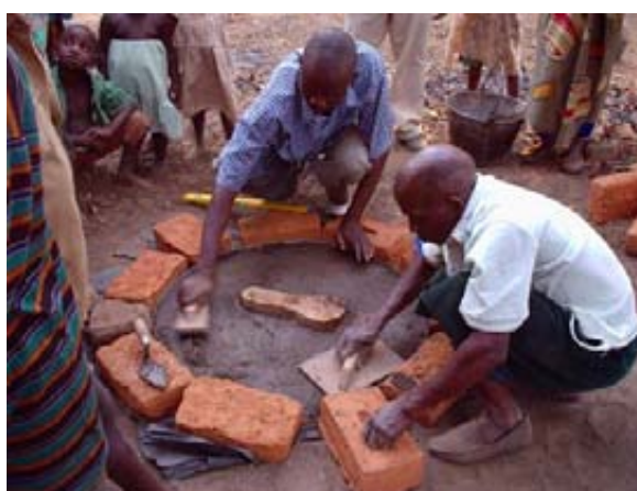
Making a round 0.8m diameter concrete slab in Malawi with sharp river sand and cement. When the river sand is of high quality, the addition of granite stones may be unnecessary. In this case a tin strip 40mm deep is formed into a circle 0.8m in diameter and supported by bricks. It is laid over a sheet of plastic. 4 wires are cut as reinforcing. In this case 2 metres of 2.5mm wire has been cut into 4 pieces (2 X 0.55m and 2 X 0.45m). 3mm or 4mm wire can also be used. The mix of sharp river sand and cement is 4 to 1(20 litres river sand and 5 litres cement). 8 slabs can be made from one 50 kg bag of cement using this method. High quality river sand and proper curing are important.
