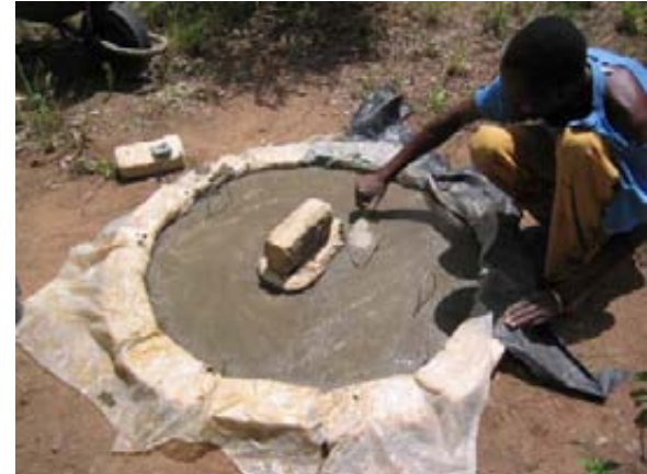
A mould for the squat hole is made with a bucket or with bricks as shown here. Half the mix (about 17 litres) is added to the mould first and levelled off. The four 90cm pieces of wire (3 – 4mm thick) are added to make a wire square around the squat hole. Then the remaining concrete is added, levelled, tamped down hard and finished off with a wooden float and steel trowel.
