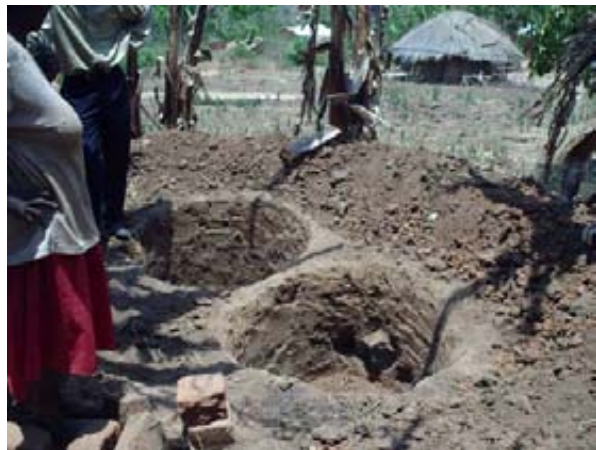
Round concrete slabs are commonly used on pit latrines in Malawi and the Fossa alterna also uses a round slab. Many of these are domed and use on reinforcing. Some are flat and use a small amount of reinforcing. The flat slab on left is 1 metre in diameter using a 3 to 1 mix of sharp river sand and cement and 2.5mm or 3mm wire as reinforcing. It is left to cure for 10 days. The twin pits are normally lined with fired bricks and bonded with traditional mortar. Photo taken in Phalombe district. On the right two pits dug prior to brick lining. Photo taken in Thyolo district. Thanks to COMWASH.
