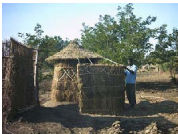
Most Arborloos in Malawi are of simple construction using poles and grass Photos taken in Embangweni (left) and Phalombe (right). Thanks to CCAP and COMWASH.
