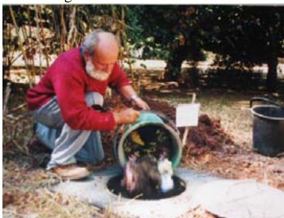
Tipping the contents of the bucket from a Skyloo into a small shallow pit for processing. The shallow pit is covered with a concrete lid with hole which is itself covered. On the left three cement jars are shown. The one actively being filled is covered with an attractive painted concrete cover.
