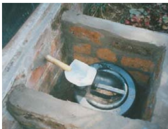
A plastic pipe is led down from the urine diverting pedestal through the side wall of the vault into a plastic container held within a small brick built side vault. A home made funnel is used to guide the urine into the container. The side vault is built up on soil so that any urine overflow can drain away.
