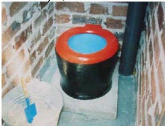
This neat and durable pedestal is constructed entirely from concrete with an internal plastic lining which is in fact a bucket. The vent pipe is fitted inside the structure. On the right, the humus from the composted vault is being removed. It was this humus that was used in the plant trials described later on in this book.
