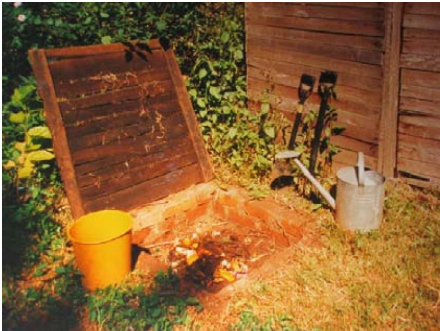
The second pit of a Fossa alterna in its first year can be used as a compost pit.
