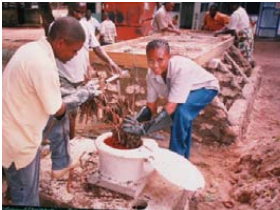
Adding semi composted palm leaves to the base of a Fossa alterna pit in Mombasa, Kenya (left). Two sacks full of leaves at the base of a concrete lined pit in Maputaland, South Africa.
