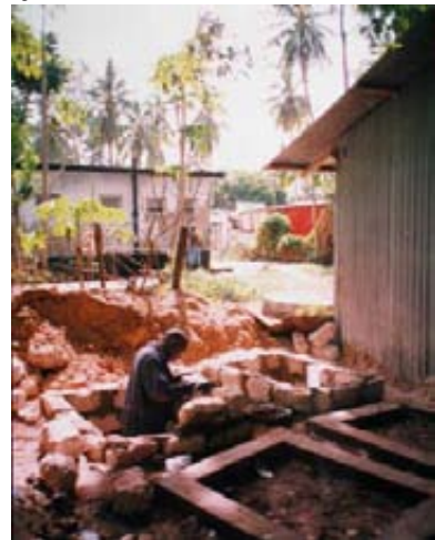
Delegates at eco-san workshop in Mombasa construct concrete ring beams within wooden frames for Fossa alterna at the Mtomondoni Primary School (left). On the right the two pits of a Fossa alterna are lined with coral limestone blocks from the base in very loose sandy soil near a beach site at Mombasa.
