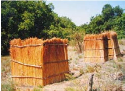
Left, the simplest superstructure – poles and grass – no door - no roof. Thanks to Jim Latham, Eco-Ed Trust. Right, slightly more advanced – pole and grass structure with door and roof. Low cost and very durable door hinges can be made with cut sections of car tyres. Photo taken an Fambidzanai – Permaculture Training Centre
