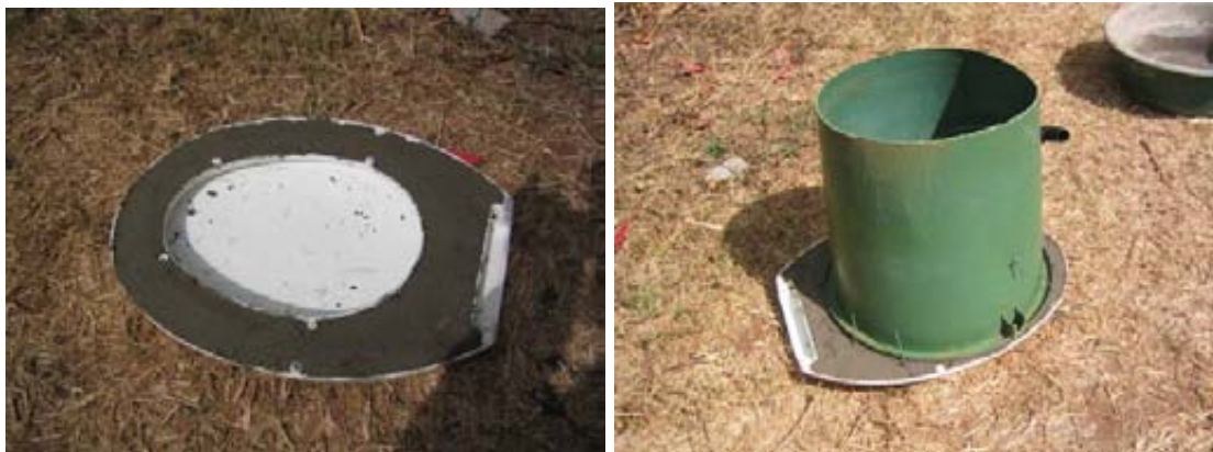
A strong mix of concrete using 3 parts river sand and 1 part cement is mixed and added to the toilet seat as shown. This will add strength to the seat and form a bond between the seat and side walls of the pedestal. The bucket is now fitted centrally over the toilet seat as shown.
