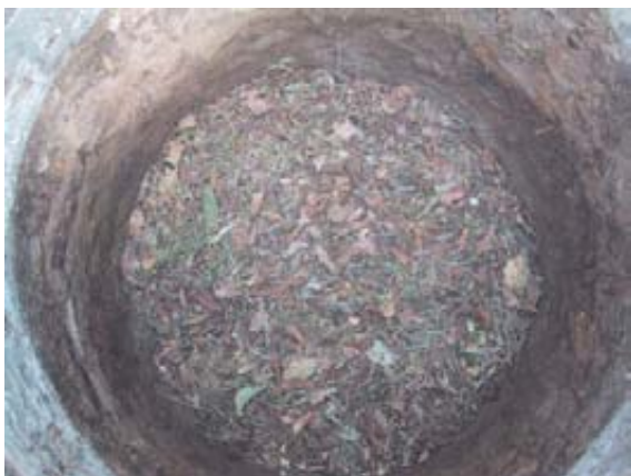
In a new series of experiments leaves are added to the bases of dug out pits and the users asked to put plenty of soil, ash and leaves into the pit as they use it. And not to use the pit as a garbage dump. It is thought that this refinement in the way pits are used will make hand excavation easy in the future. Where twin pits are used, the family alternates the use from one pit to the other. The pits under investigation are lined with concrete rings. Each concrete ring is 1m in diameter and 40cm deep. Up to 6 rings are used to line a pit. Pits of this size (1.8 cu.m.) can last a family up to 5 years.
