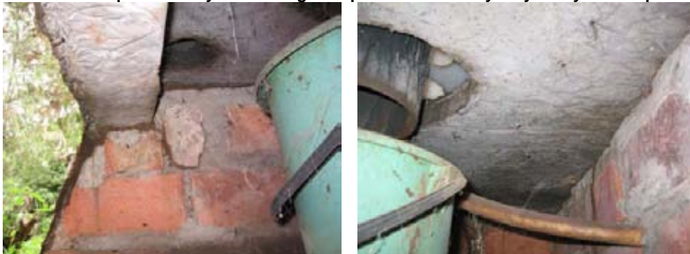
Flies have never been seen in the Skyloo system, but spiders and mosquitoes do invade during the wet season. Spiders do no harm but can block vent pipes. Mosquitoes in this case are the culix type and not malaria carrying. They look for dark places to hide – they do not breed there – there is no water.
