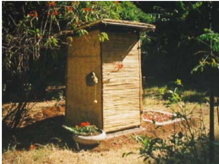
The Fossa alterna is designed to make humus from human excreta. It has two shallow pits protected by two concrete ring beams, a single concrete slab and a superstructure, in this case made from gum poles and reed mats. This unit is also equipped with a low cost home-made pedestal, a vent pipe and hand washing device. The system is simple and can be made at low cost. Photo taken in Marlborough, Harare.
