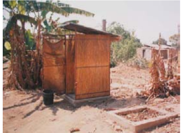
Fitting the portable superstructure to one of the twin Fossa alterna pits in Epworth, close to Harare. During the first year the second pit was filled with leaves and thin layers of soil to make leaf mould. After 12 months the leaf mould was dug out and the slab and structure moved to the second pit (as shown). The pit filled with excreta, soil, ash and leaves has been topped up with soil (see right of picture).
