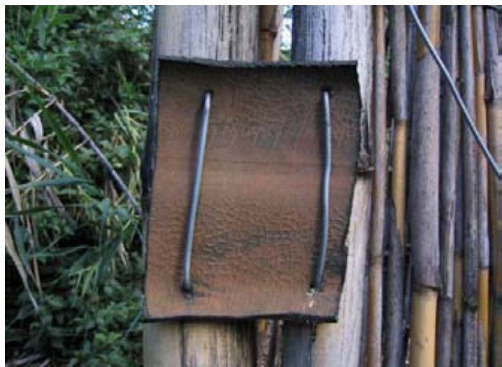
Structure made of bamboo and reeds. The four main bamboo uprights are anchored in the ground. They can be protected to a certain extent from ants with old engine oil or wood ash. The hinge for the door is made of old car tyre, as shown on the right. This material makes an effective and durable hinge.
