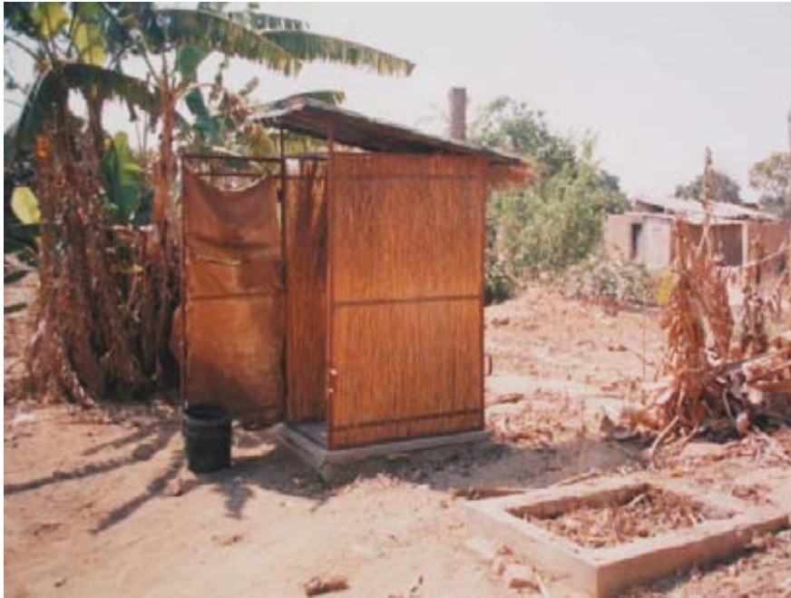
A Fossa alterna in Epworth, Zimbabwe. The twin pit system makes humus
