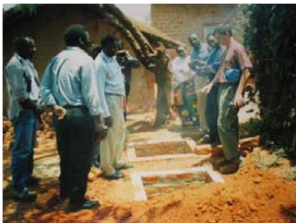
On the left two brick ring beams have been built for a Fossa alterna in Lichinga, Niassa Province Mozambique. On the right two brick ring beams have been built in Kusa, near Kisumu, Kenya. The ring beams are permanently sited and are best bonded with strong cement mortar.
