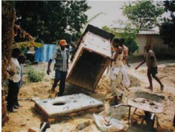
Fitting the portable superstructure to one of the twin Fossa alterna pits in Epworth, close to Harare. During the first year the second pit was filled with leaves and thin layers of soil to make leaf mould. After 12 months the leaf mould was dug out and the slab and structure moved to the second pit (as shown). The pit filled with excreta, soil, ash and leaves has been topped up with soil (see right of picture).
