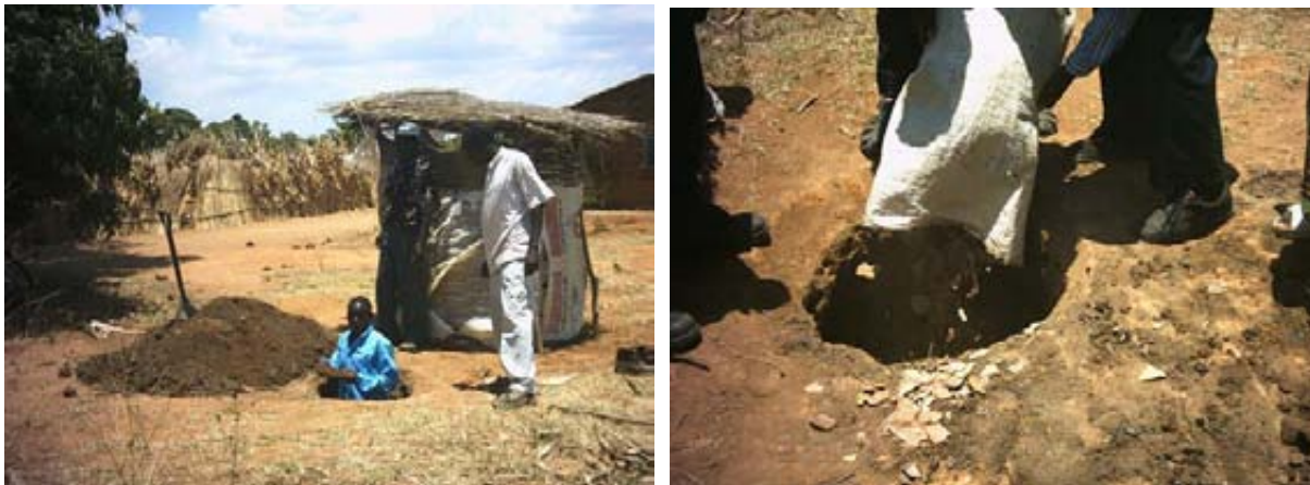
Excavation of Fossa alterna pit in Embangweni. In this case the structure is a simple bamboo portable unit which is moved from one pit the other. The ground is very firm in this locality and no ring beam or pit lining was used. The pit took less than 30 minutes to excavate and the entire operation of excavating and moving the slab and structure to the newly excavated pit took less than one hour. On the right dried leaves are being placed down the new pit. These help to compost the excreta like the soil which is added.
