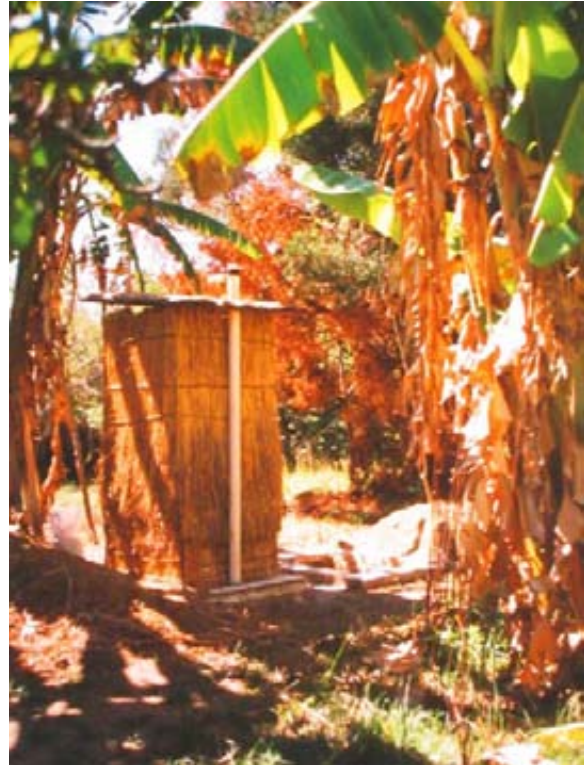
On the left the prototype Fossa alterna used a wooden structure and two shallow pits with brick ring beams. On the right a Fossa alterna in a low density suburb in Harare. This unit used two concrete ring beams, a structure made with a steel frame overlaid by grass and a 75mm PVC vent pipe.
