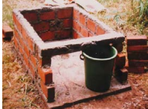
Stages in making the vault. The brickwork
