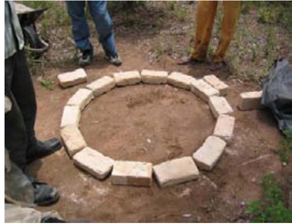
The circle for the 1 metre diameter slab mould is marked on levelled ground and bricks placed together in a circle
