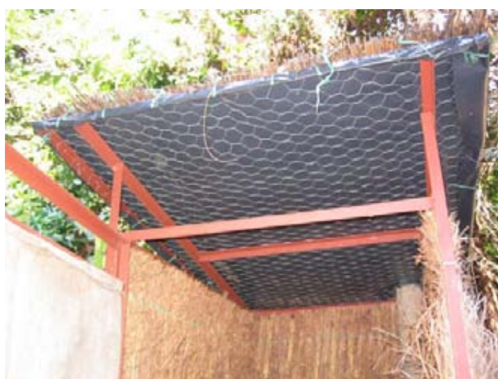
Close up of upper parts of the frame and roof
