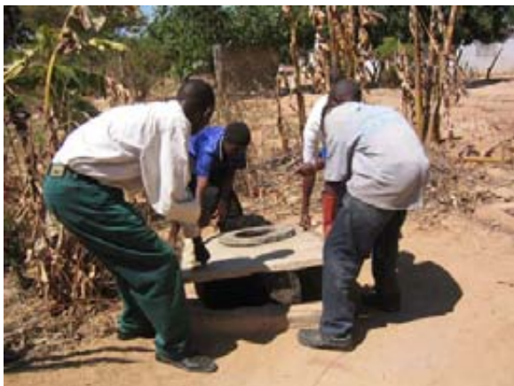
The concrete slab is now removed using the four handles and this is immediately placed over the now empty pit nearby. The slab is levelled and best laid on a bed of weak cement mortar laid over the pit lining brickwork.
