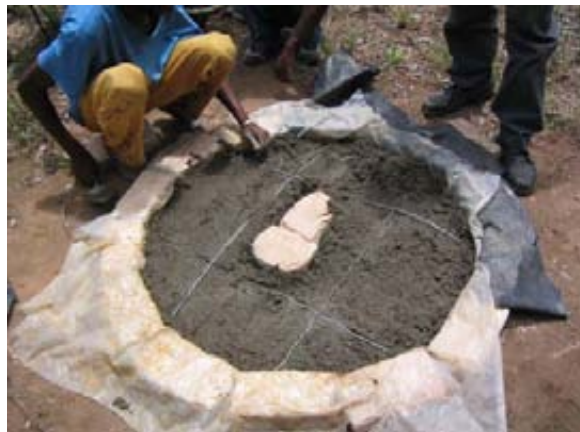
A mould for the squat hole is made with a bucket or with bricks as shown here. Half the mix (about 17 litres) is added to the mould first and levelled off. The four 90cm pieces of wire (3 – 4mm thick) are added to make a wire square around the squat hole. Then the remaining concrete is added, levelled, tamped down hard and finished off with a wooden float and steel trowel.
