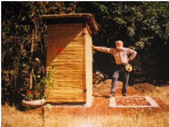
Fossa alterna at Woodhall Road, Harare. Note hand washing facility, waste water falling into a flower pot. Second pit during the first year was filled with leaves and compost. It was also used to grow comfrey (see later). Inside a home made pedestal has been fitted. The yellow bucket contains a mix of soil and wood ash and a dispenser. Leaves are also added occasionally.
