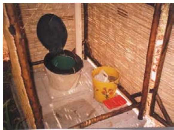
Fossa alterna at Woodhall Road, Harare. Note hand washing facility, waste water falling into a flower pot. Second pit during the first year was filled with leaves and compost. It was also used to grow comfrey (see later). Inside a home made pedestal has been fitted. The yellow bucket contains a mix of soil and wood ash and a dispenser. Leaves are also added occasionally.
