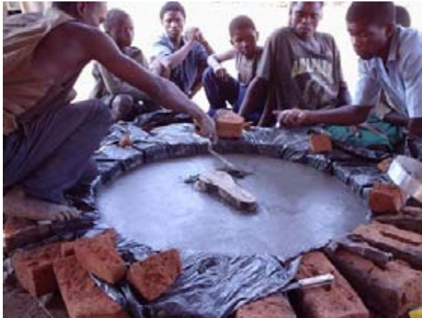
Round concrete slabs are commonly used on pit latrines in Malawi and the Fossa alterna also uses a round slab. Many of these are domed and use on reinforcing. Some are flat and use a small amount of reinforcing. The flat slab on left is 1 metre in diameter using a 3 to 1 mix of sharp river sand and cement and 2.5mm or 3mm wire as reinforcing. It is left to cure for 10 days. The twin pits are normally lined with fired bricks and bonded with traditional mortar. Photo taken in Phalombe district. On the right two pits dug prior to brick lining. Photo taken in Thyolo district. Thanks to COMWASH.
