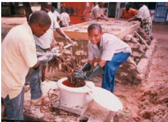
On the left adding semi-composted "makuti," the leaf of the palm tree, to the base of a Fossa alterna to promote composting. On the right a finished Fossa alterna at Bengala Village. Both pits, dug down to 1.5m are fully lined with coral limestone blocks in loose soil. The second pit has been left empty and covered with a tin lid. The addition of soil, wood ash and leaves to excreta promotes composting in the pits. It is this promotion of the composting process which makes the Fossa alterna concept possible.
