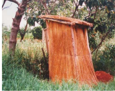
Left, the simplest superstructure – poles and grass – no door - no roof. Thanks to Jim Latham, Eco-Ed Trust. Right, slightly more advanced – pole and grass structure with door and roof. Low cost and very durable door hinges can be made with cut sections of car tyres. Photo taken an Fambidzanai – Permaculture Training Centre
