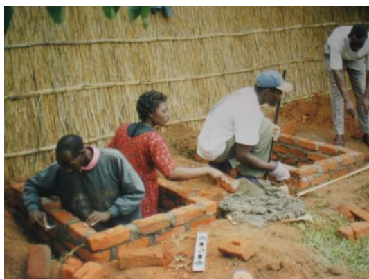
Fossa alterna ring beams being constructed in Lilongwe, Malawi. Here the soil is firm. In this case the pit is first dug down to about one metre. The upper end has then been widened to allow for the 2 course brick ring beam to be constructed from one brick course below ground level. Two brick courses have been built above ground level. Soil taken from the pits is then built up around the two ring beams. This raises the site of the toilet above the surroundings, which helps divert rainwater from the site.
