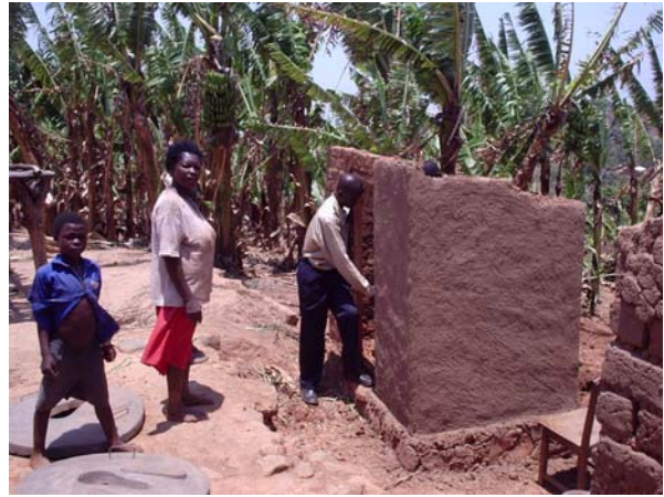
On the left a grass structure for the Fossa alterna in Salima district. Both pits are placed within the superstructure. On the right a permanent brick structure is built over two pits lined with bricks in Thyolo.
