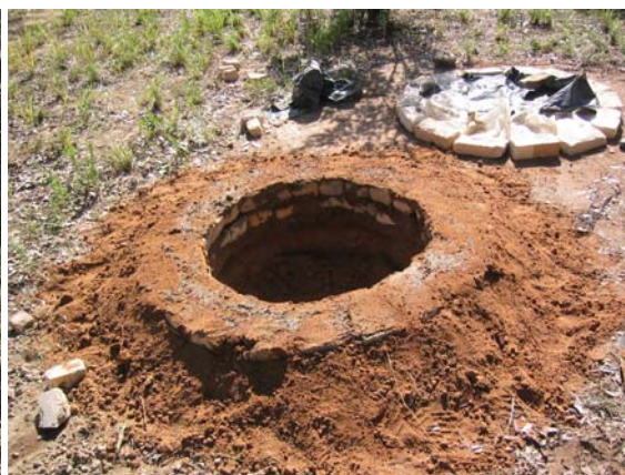
The pit is dug out down to 1 – 1.5 metres and the extracted soil placed around the ring beam and rammed in place. The ring beam and surrounding soil will help to make the toilet stable.
