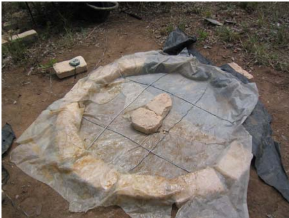
Plastic sheet is placed inside the mould and the concrete mix is made up in a wheel barrow (30 litres of good clean river sand and 5 litres of fresh cement). This is thoroughly mixed before and after adding water to make the concrete mix. Using this economy mix 8 slabs can be made with a single 50kg bag of cement.
