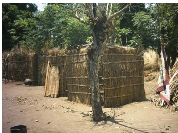
Simple grass superstructure for the Fossa alterna on the left in Njerema Village, Salima. On the right a view through the entrance showing one pit covered with a squatting slab and the second pit awaiting a cover. The Fossa alterna pits in loose sandy soils are lined from the bottom with bricks. Thanks to WaterAid.
