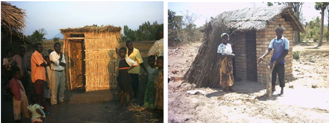
Simple eco-toilets in Malawi. On the left an Arborloo , on the right a Fossa alterna
