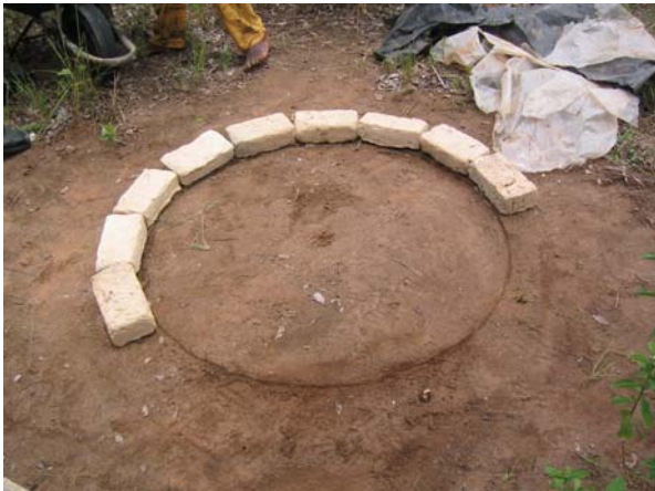
The circle for the 1 metre diameter slab mould is marked on levelled ground and bricks placed together in a circle
