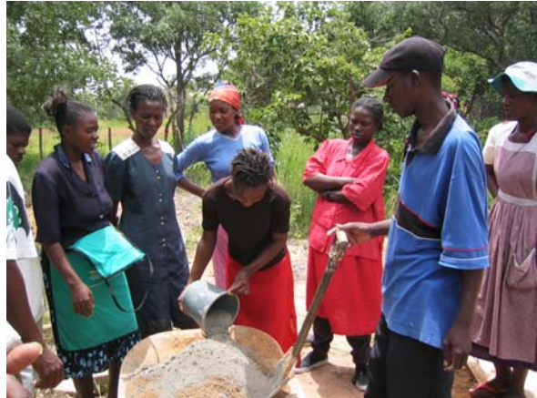
Plastic sheet is placed inside the mould and the concrete mix is made up in a wheel barrow (30 litres of good clean river sand and 5 litres of fresh cement). This is thoroughly mixed before and after adding water to make the concrete mix. Using this economy mix 8 slabs can be made with a single 50kg bag of cement.
