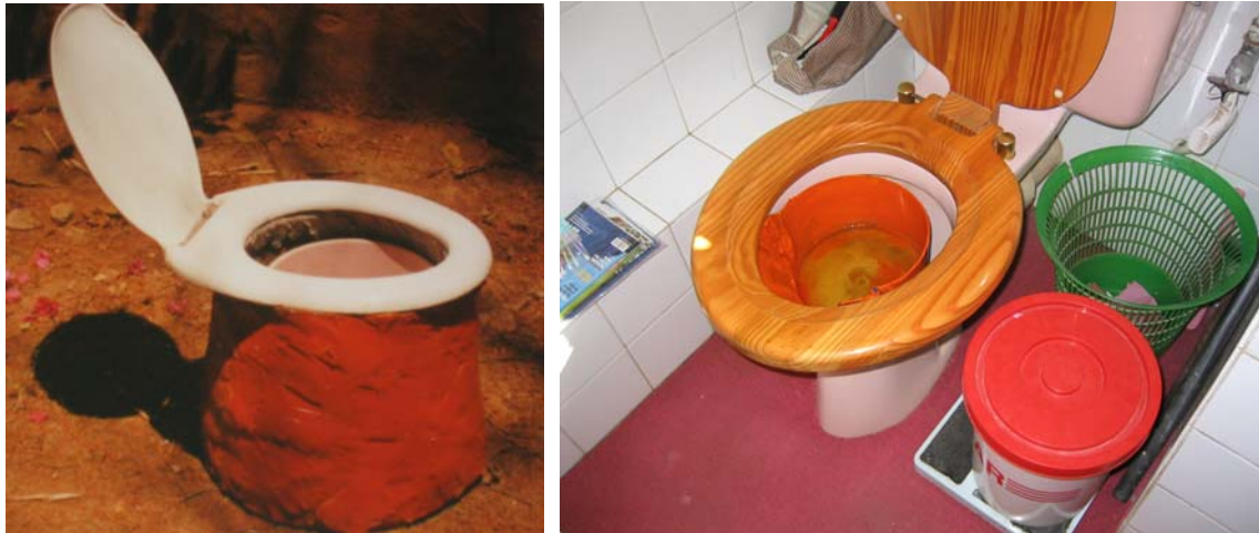
On the left a 10 litre bucket is placed beneath a pedestal which helps women to collect urine. On the right a urine collector shaped from a plastic bucket is used to collect urine from a standard flush toilet.
