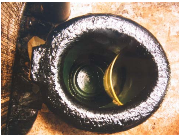
On the left the completed urine diverter fitted to a Skyloo. The bucket which collects the faeces, soil and ash can be seen directly beneath the pedestal. On the right a home made urine diverting pedestal made in Kenya.
