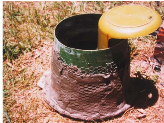
Stages in making one “home made version” of a urine diverting pedestal. Urine in this case ran down through the hole into another plastic bucket held within the vault and then to a soakaway.
