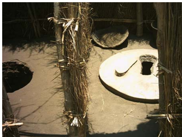
Simple grass superstructure for the Fossa alterna on the left in Njerema Village, Salima. On the right a view through the entrance showing one pit covered with a squatting slab and the second pit awaiting a cover. The Fossa alterna pits in loose sandy soils are lined from the bottom with bricks. Thanks to WaterAid.
