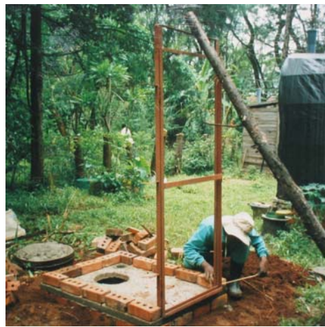
One of the two pits is dug and lined with cement mortared fired bricks. The steel frame (with door frame) is erected at the “door” end of the slab and the brick walls are built. “Sprags” of steel welded to the frame link the steel component with the brick and mortar work.
