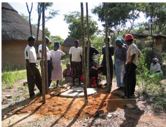
The slab is then moved and placed over the ring beam embedded in a layer of anthill mortar to keep it steady. The superstructure is now built with locally available materials like wooden poles and grass).
