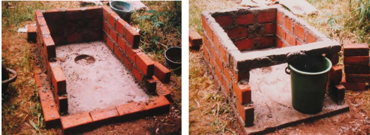
Stages in making the vault. The brickwork
