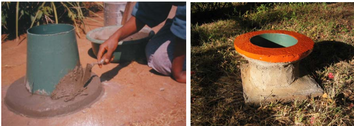
Very low cost pedestal made from a ten litre plastic bucket and cement only. It is durable and with suitable painting can be made very smart.
