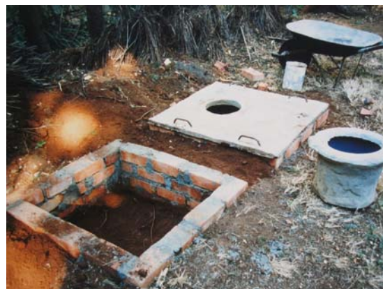
The concrete slab is bedded into a layer of weak cement mortar on the ring beam. The photo on the left shows one being fitted at Epworth. The photo on the right shows the prototype fitted in Woodhall Road. Carrying handles are useful when moving the slab from one pit to the other
