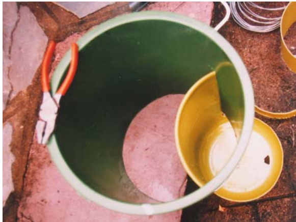
Stages in making one “home made version” of a urine diverting pedestal. Urine in this case ran down through the hole into another plastic bucket held within the vault and then to a soakaway.
