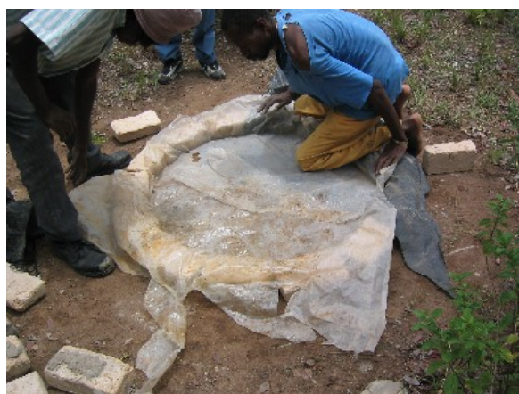
The squat hole is made by placing a shaped plastic bucket or shaped bricks in the slab mould.
