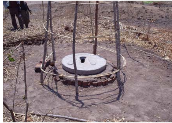
Another case in Malawi showing corbelled brickwork protecting a shallow pit of an Arborloo . Once again the diameter of both the pit and slab is 0.6m. Here the poles for the structure have been mounted in the ground before soil from the pit soil is placed back around the brickwork up to slab level.
