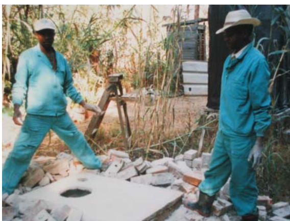
All the brickwork has been taken apart. The bricks are cleaned up. This is easy because the mortar is weak (20:1 sand and cement). On the right the same slab, having been removed from the original pit, is relocated on the second pit and mounted over a bed of weak cement mortar.
