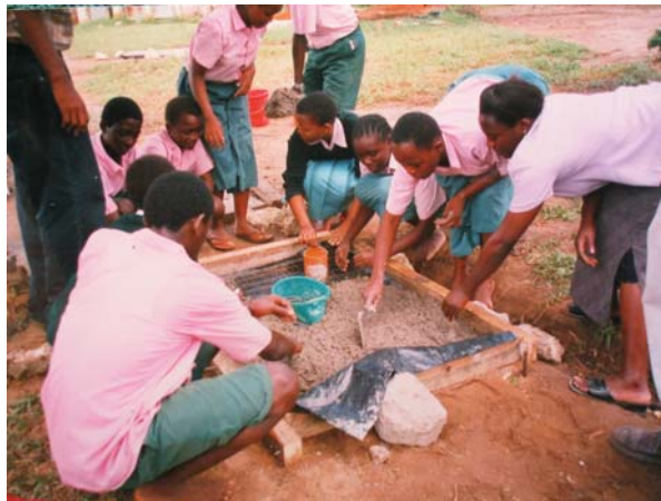
School children at the Mtomondoni Primary School learn how to make concrete slabs for eco-toilets
