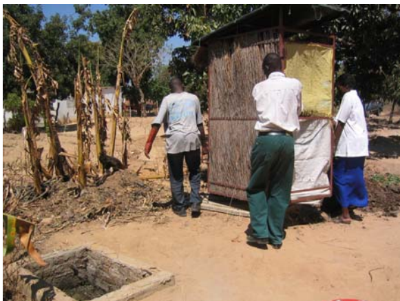
Finally the superstructure (with pedestal and vent pipe in this case) is placed over the slab. The toilet can now be put to use immediately. On the right the pit used during the previous 12 months is not yet full, but a 12 month cycle of change is easy to remember. The pit contents are now covered with a generous layer of leaves and then topsoil is added. The mixed contents of the pit are then allowed to make compost for a further 12 months, while the used pit fills up again with a mix of ingredients. The whole process is then repeated every year. With this technique the pits are re-used repeatedly and every year a valuable supply of humus is produced. It is a simple technique which has great value.
