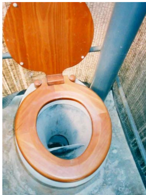
On the left the home made urine diversion unit is fitted over the slab. On the right the improved urine diverting pedestal, fitted with wooden seat. Note also the vent pipe fitted behind the pedestal to the right.
