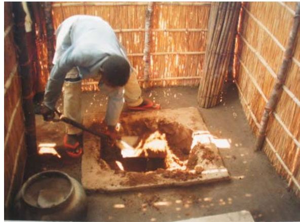
Fossa alterna in Niassa Province, Mozambique built under the WaterAid funded programme. The twin pits are enclosed in a single pole and grass superstructure which is permanently located. A washing area is also constructed as part of the system. These are very popular units, as they are almost odour and fly free, unlike many earlier toilets built in the area. They are also relatively low cost. The pits are each 1.5 metres deep and protected by brick ring beams. Here one of the pits is being excavated for humus.
