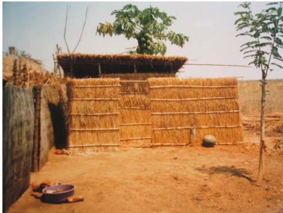
Fossa alterna in Niassa Province, Mozambique built under the WaterAid funded programme. The twin pits are enclosed in a single pole and grass superstructure which is permanently located. A washing area is also constructed as part of the system. These are very popular units, as they are almost odour and fly free, unlike many earlier toilets built in the area. They are also relatively low cost. The pits are each 1.5 metres deep and protected by brick ring beams. Here one of the pits is being excavated for humus.
