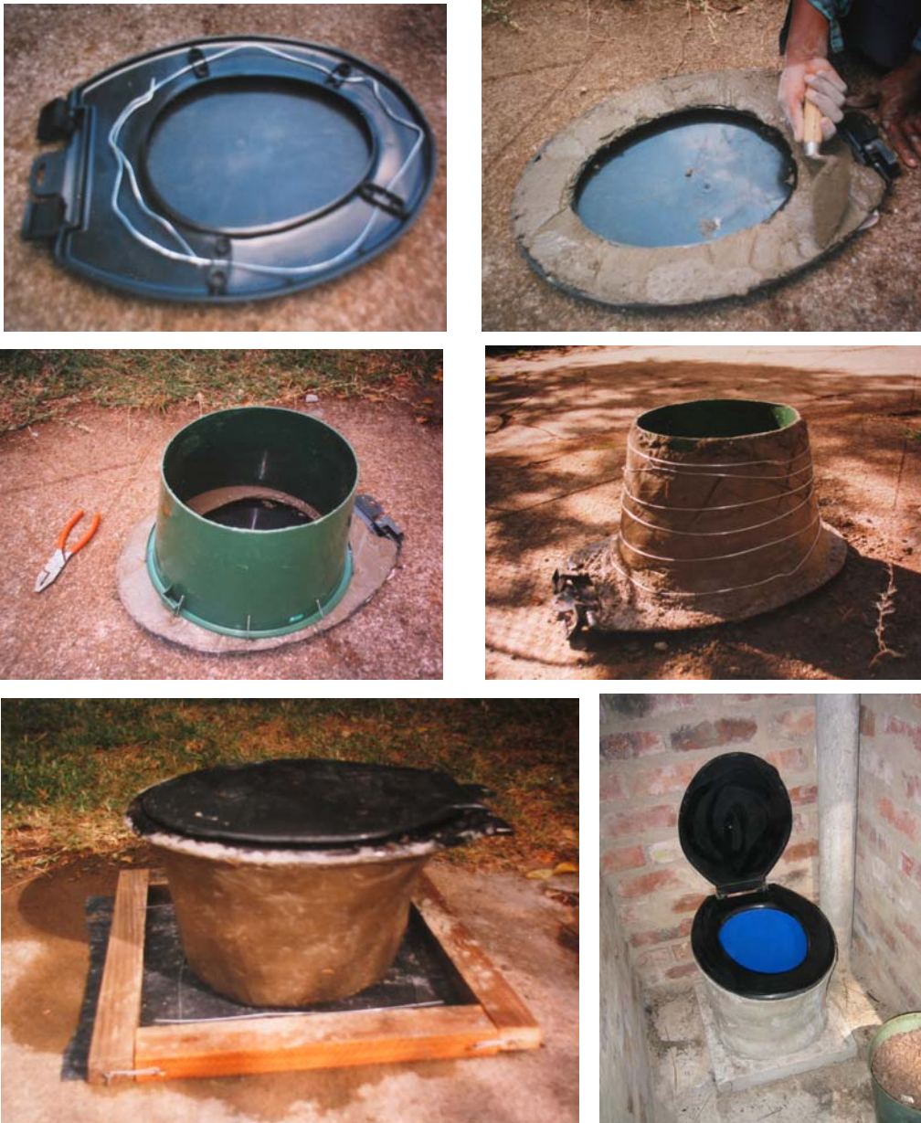
Finally a strong durable pedestal is made
