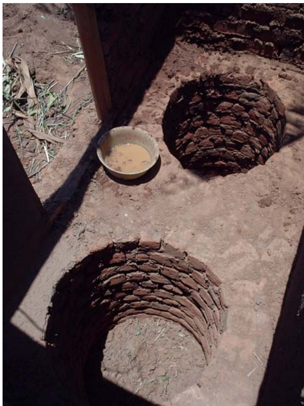
The interior of the structure shown above on right showing the two brick lined pits within the brick structure. On the left a demonstration structure showing one pit covered with a squatting slab and the other covered with a plain slab. Photo on left taken in Thyolo, photo on right taken in Phalome. Thanks to COMWASH
