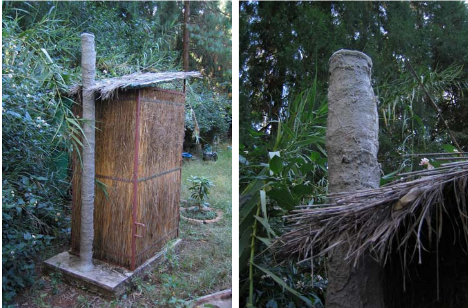
A durable home made vent pipe constructed from Hessian and a sand cement slurry with some wire reinforcing. Very effective and longlasting.
