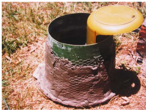
In this method the urine diverter (yellow) is made from a 10 litre bucket and fitted inside the larger chute bucket (25 litre) with wire straps. These wires pass through the plastic and later cement work. The rest of the pedestal is then built up as described earlier. A plastic pipe fitting is then attached to the yellow bucket to lead the collected urine into a urine storage vessel.
