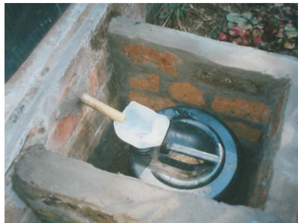
A plastic pipe is led down from the urine diverting pedestal through the side wall of the vault into a plastic container held within a small brick built side vault. A home made funnel is used to guide the urine into the container. The side vault is built up on soil so that any urine overflow can drain away.
