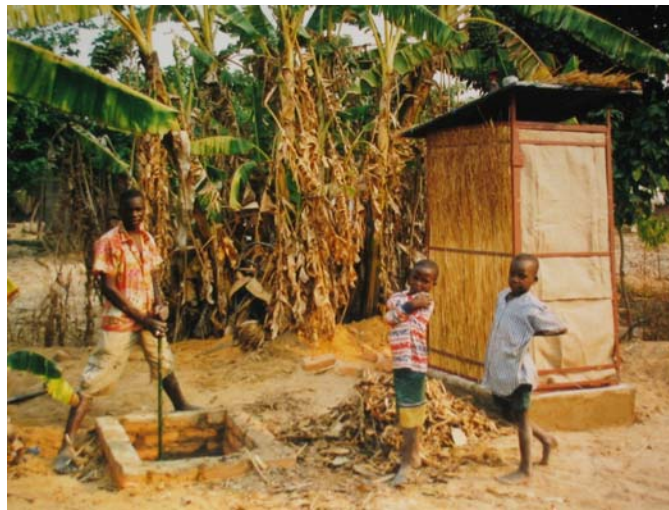
Fossa alterna in Epworth near Harare. It has two shallow pits, a single concrete slab and single superstructure, made with a light steel frame covered with grass. The Fossa alterna was initially designed for per-urban use on medium sized plots, but can be used on smaller plots and also in the rural areas.
