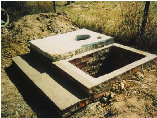
The strongly built double vault substructure is built up to about two courses above ground level. The dividing wall is a double thickness of bricks and should be plastered on either side. Once the slab is mounted, a specially designed “easy to dismantle” brick superstructure is built (see above). During the first year, the second vault can be filled with leaves and soil to make leaf mould.
