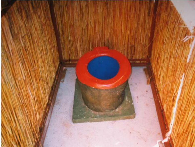
Home made pedestal placed on the slab. The pedestal is smart, cheap and durable.
