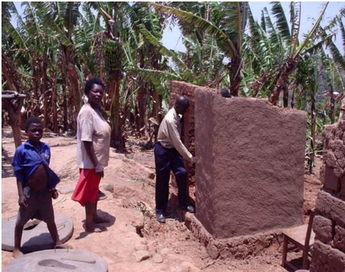
On the left a permanent brick Fossa alterna structure is built around two brick lined pits in Thyolo, Malawi (COMWASH Project). The brick lined pits are shown on the right.
