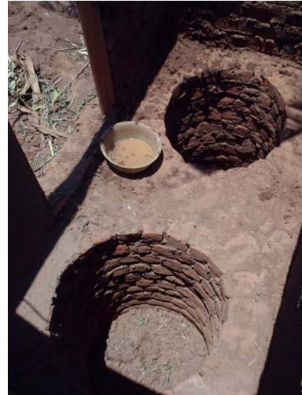
On the left a permanent brick Fossa alterna structure is built around two brick lined pits in Thyolo, Malawi (COMWASH Project). The brick lined pits are shown on the right.
