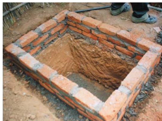
Fossa alterna ring beams being constructed in Lilongwe, Malawi. Here the soil is firm. In this case the pit is first dug down to about one metre. The upper end has then been widened to allow for the 2 course brick ring beam to be constructed from one brick course below ground level. Two brick courses have been built above ground level. Soil taken from the pits is then built up around the two ring beams. This raises the site of the toilet above the surroundings, which helps divert rainwater from the site.
