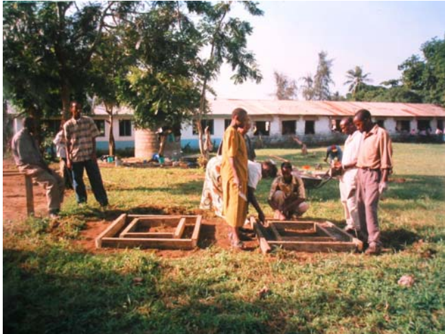
Delegates at eco-san workshop in Mombasa construct concrete ring beams within wooden frames for Fossa alterna at the Mtomondoni Primary School (left). On the right the two pits of a Fossa alterna are lined with coral limestone blocks from the base in very loose sandy soil near a beach site at Mombasa.
