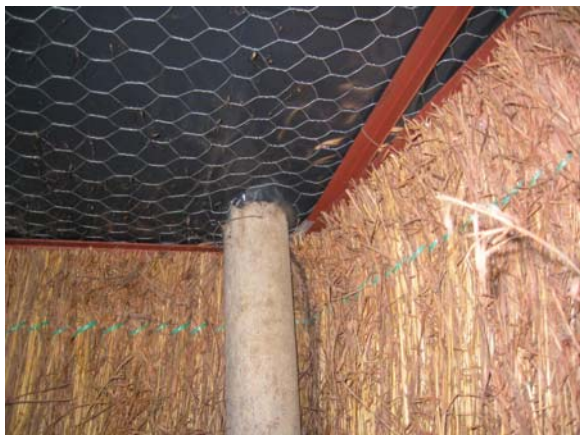
The asbestos pipe passing through the roof and a neat seat made from a bucket and concrete work only.
