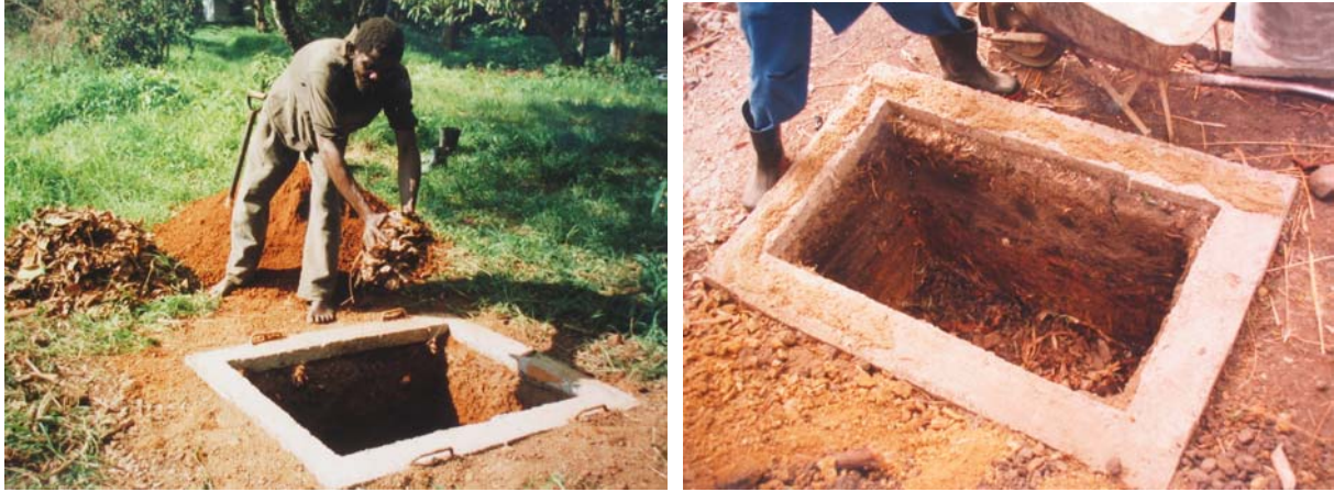
Adding dry leaves to the base of a pit helps the composting process. A full sack full or even two sacks full works well. The pit is ready – ring beam in place and leaves at bottom.
