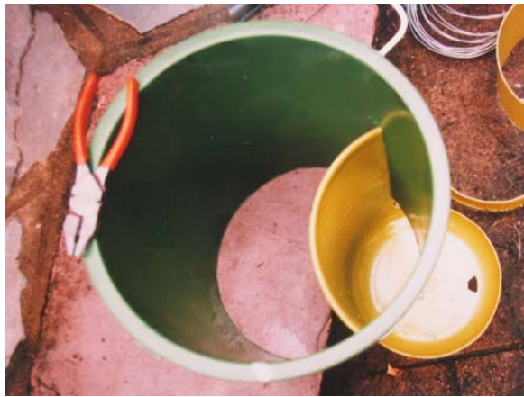
In this method the urine diverter (yellow) is made from a 10 litre bucket and fitted inside the larger chute bucket (25 litre) with wire straps. These wires pass through the plastic and later cement work. The rest of the pedestal is then built up as described earlier. A plastic pipe fitting is then attached to the yellow bucket to lead the collected urine into a urine storage vessel.
