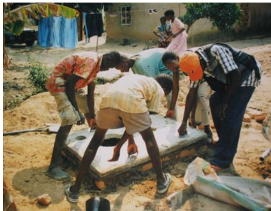
The concrete slab is bedded into a layer of weak cement mortar on the ring beam. The photo on the left shows one being fitted at Epworth. The photo on the right shows the prototype fitted in Woodhall Road. Carrying handles are useful when moving the slab from one pit to the other
