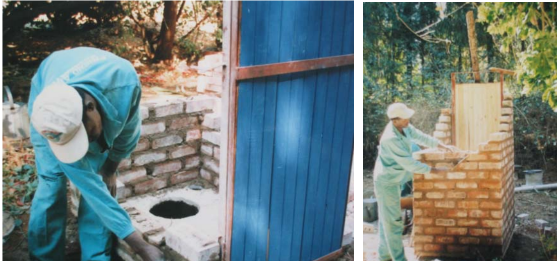
The steel frame is mounted again on the slab and the same bricks are used to rebuild the structure.
