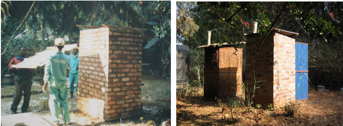
After the brickwork is complete, the roof, asbestos pipe and pedestal can be put back in place. The operation takes about 6 hours. If the pits are changed once every 3 – 5 years, this is not a huge expenditure of time and effort. Everything is recycled, even the material in the pit, which is dug out once the time has come to change sides again.
