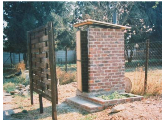
The strongly built double vault substructure is built up to about two courses above ground level. The dividing wall is a double thickness of bricks and should be plastered on either side. Once the slab is mounted, a specially designed “easy to dismantle” brick superstructure is built (see above). During the first year, the second vault can be filled with leaves and soil to make leaf mould.
