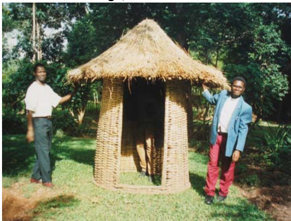
Woven basket superstructure from Malawi. Thanks to Steven Sugden and WaterAid. Woven basket structure on Arborloo in Northern Malawi. The door is made from sacking. A neat and effective unit. Photo: thanks to Jim McGill, Embangweni eco-san project.
