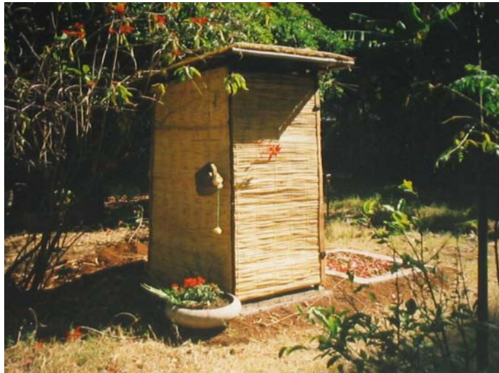
The Fossa alterna is designed to make humus from human excreta. It has two shallow pits protected by two concrete ring beams, a single concrete slab and a superstructure, in this case made from gum poles and reed mats. This unit is also equipped with a low cost home-made pedestal, a vent pipe and hand washing device. The system is simple and can be made at low cost. Photo taken in Marlborough, Harare.
