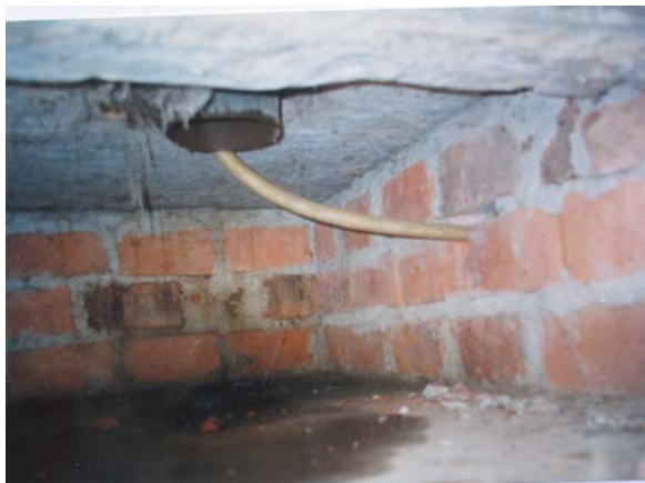
A plastic pipe is led down from the urine diverting pedestal through the side wall of the vault into a plastic container held within a small brick built side vault. A home made funnel is used to guide the urine into the container. The side vault is built up on soil so that any urine overflow can drain away.
