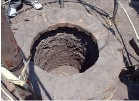
Another case in Malawi showing corbelled brickwork protecting a shallow pit of an Arborloo . Once again the diameter of both the pit and slab is 0.6m. Here the poles for the structure have been mounted in the ground before soil from the pit soil is placed back around the brickwork up to slab level.
