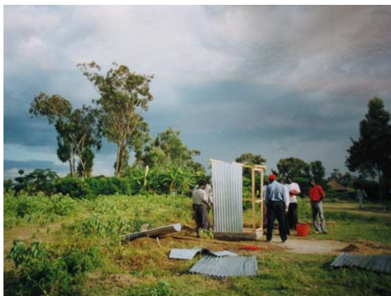
On the left a Fossa alterna with portable structure being constructed in Kusa Village, Kisumu, Kenya. On the right a permanent brick and thatch Fossa alterna built at Kufunda Village, Ruwa, Zimbabwe
