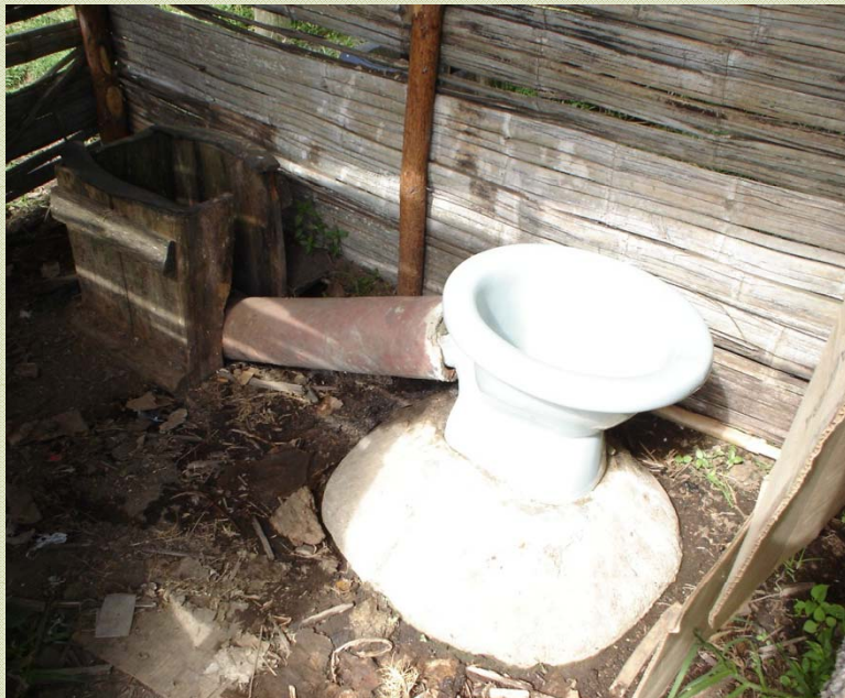
Abandoned bucket-flushed toilet
