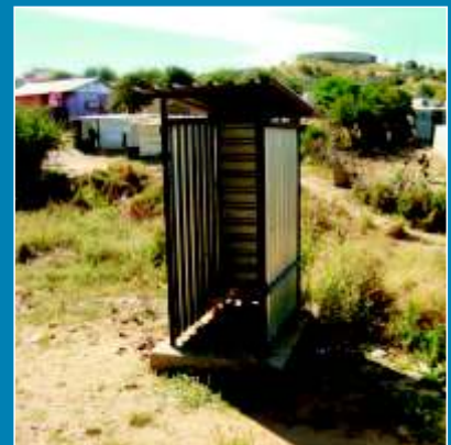
A vandalised enviroloo toilet in Katutura informal settlements, Windhoek
