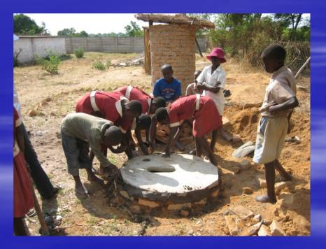
At this stage we have a fully brick lined pit which is stable and a strong concrete slab capping the pit fitted with a squat and ventilation pipe hole.
