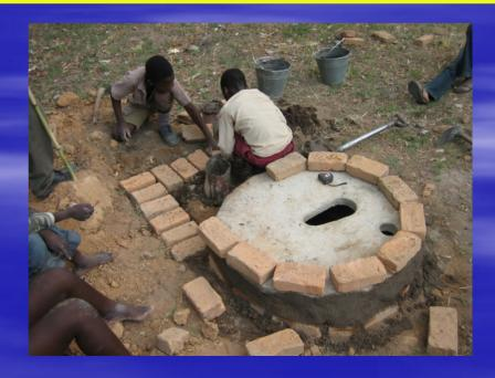
The foundations are built up using weak cement mortar (16:1) to the level of the slab. We can see the shape building up. Bricks mounted on the slab itself are shaped in a circle. The photo on the right shows the first layer of superstructure brickwork. The space between the wall and slab is filled with soil and compacted.
