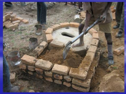
The superstructure walls are then built up with 19 courses of bricks. At about the 15th course a series of glass bottles are introduced into the wall of the structure to allow a little more light into the Blair VIP.
