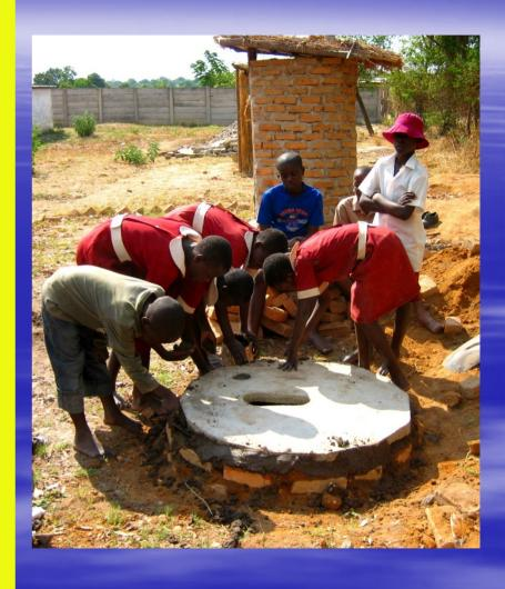
In this case we shall show how a spiral bricked walled Blair VIP can be made. This is made without a door and has no moving parts which can wear out (just like the standard Blair VIP). With the spiral version of the Blair VIP part of the superstructure is built off the slab and to one side. It is important to build a brick foundation on which the brick wall will be mounted outside the slab.
