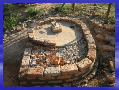
The extension of the slab and toilet floor outside the slab area for the spiral superstructure
