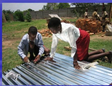
The three iron sheets are laid over the roof timbers so that it is completely covered. Nails are then used to secure the sheets to the wooden frame.
