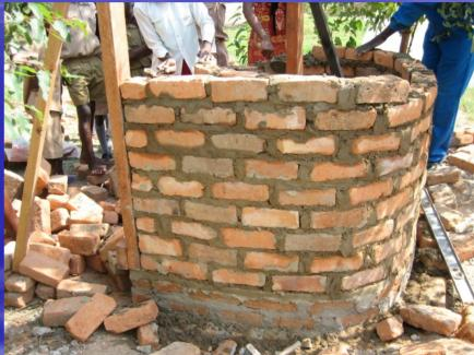
The spiral shape of the structure provides great strength to the wall, even if it not made perfectly.
