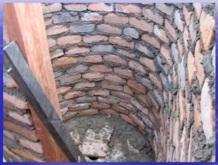
This special design with its curved 6 or 9 shape follows the rim of the slab for most of its length making it easier to build for pupils. The wall follows a well defined line of construction. The shape – full of curves provides a natural structural strength. The use of templates also assists by defining the ends of the curved wall with vertical guides. These special features of this design make the larger and more universal spiral BVIP easier to build.
