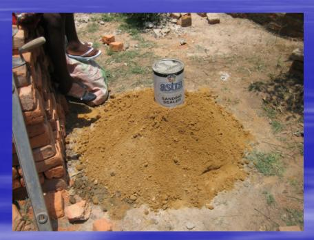
About 400 – 500 burnt pricks are required for the spiral superstructure. The mortar mix is 20 parts pit sand and 1 part cement (PC15 – Portland).
