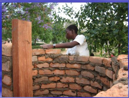
Traditional mortar can also be used to bond the brickwork. 2 parts sandy soil and 1 part termite hill soil
