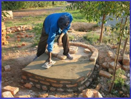
The final result at this stage is a flat surface on which the spiral superstructure can be built. The extension of the slab is about 65cm.
