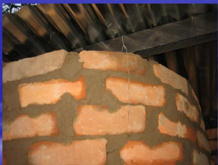
The wires are placed around the wooden frame and through the brickwork mortar 3 courses down from the top.
