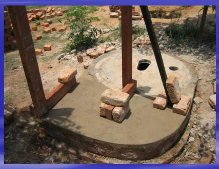
The specially designed wooden templates are placed on the slab as shown. Using a spirit level both are made vertical. Each templates acts as a guide to the end of the brick wall. Note the orientation of the squat hole towards the spiral opening.
