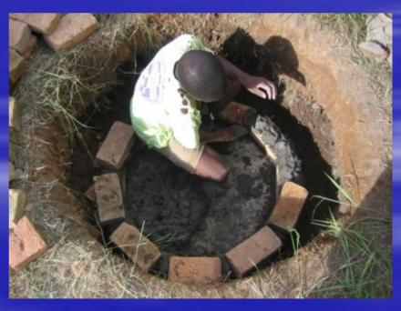
The walls of the tank are built up to at least one course above ground level. The wall carrying the PVC pipe from inside the urinal should be above this level to maintain the slope.
