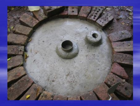
Inside the urinal the PVC pipe is made to fit the wall closely. Outside the urinal the tank cover has been fitted and the PVC pipe positioned to run into the centre hole with the screen
