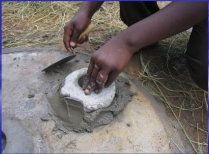
The final installation. The PVC Blair Pump (mini version) has been fitted. A small concrete apron is laid down where the bucket which collects urine will be placed.
