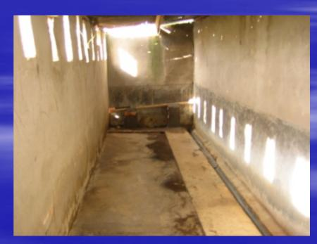
The PVC pipe is secured in place. A special concrete fitting is made with the threads of the pump cast into it. The PVC pump (a small version of the Blair Pump) as a thread on it which screws into the thread held in the concrete casting.
