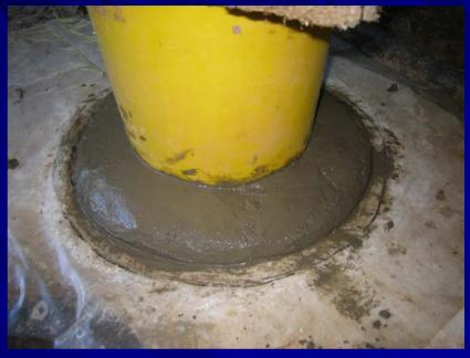
A mix of cement and river sand is now made up. If Portland cement is used the mix is 1 part cement and 3 parts river sand. If masonry cement is used a 1:1 mix is used. The concrete can be mixed in small lots with a litre of cement being mixed with the sand at any one time. The concrete is made into a neat round shape with a trowel. A ring of 3mm wire is placed inside the concrete.
