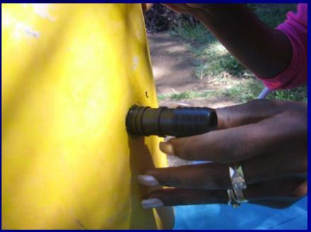
The hole must be cut precisely so the plastic pipe fits tight.
