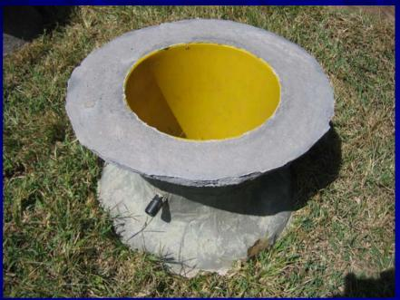
It is important that the concrete work be allowed to cure fully to gain maximum strength. After this period the pedestal is placed in the sun and allowed to dry out completely.
