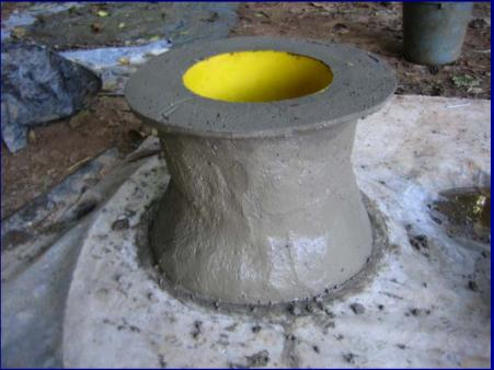
The base of the pedestal is built up in the same way using the same mark on the plastic sheet. A 3mm wire ring is placed in the concrete. The concrete is shaped neatly so that upper and lower layers meet to form a strong shell around the bucket. The pedestal is then covered with plastic sheet. The next day it is watered and kept wet for at least 7 days to cure.
