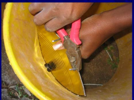
Wires are then used to secure the tin in position. The wires are bent over the tin sheet.
