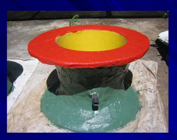
After this the concrete can be painted with brightly coloured enamel paint. The unit will still work if not painted, but is more attractive if brightly coloured. The urine pipe placed above slab level makes it possible to divert the urine to a tree or plastic container even when the toilet is placed over a pit.
