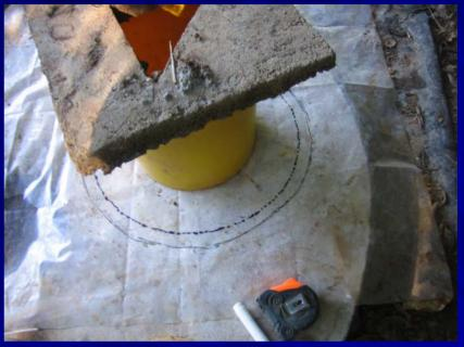
A 10 litre plastic bucket is used and the base sawn off. The bucket is placed base down on a piece of clear plastic and a mark drawn 75cm around the bucket. To keep it secure a weight is placed on top of the bucket.
