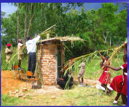
This is a round structure with a door. But durable and low cost structures can be built without a door like the "old" Blair VIP!.
