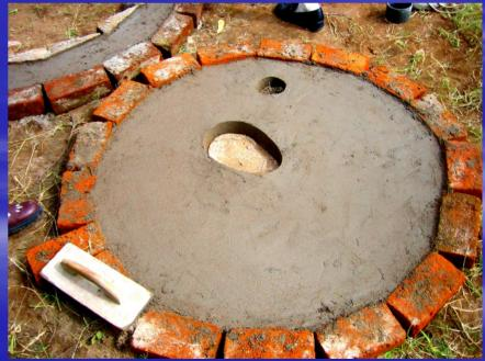
Where the ground is moderately firm and there are no bricks available a "ring beam" can be used to protect the pit.
