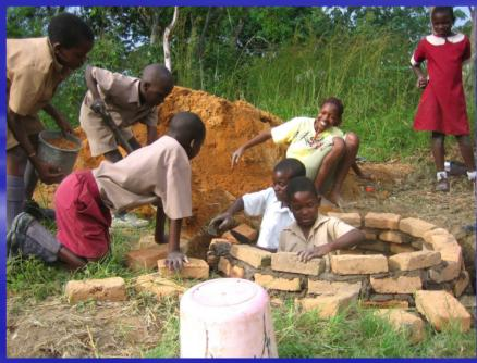
Once the concrete slab is laid (in mortar) on top of the lined pit a wide range of superstructures can be built on top.
