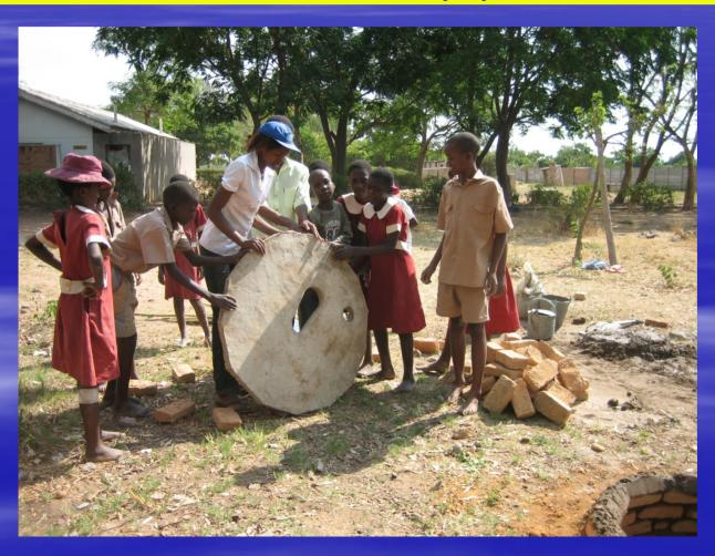
The concrete slab is quite easy to make once the training has taken place. A 1.1metre diameter slab uses 10 litres of cement and 50litres of river sand and about 8m of 3mm wire. A full bag of cement holds 50 litres of cement.
