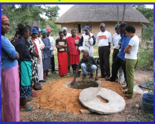
But concrete slabs which can be used on a range of "upgradeable" toilets including the Blair VIP must have a hole made to fit a ventilation pipe
