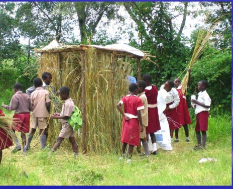
The "ring beam method" is fast, low cost and simple, but the pit is small and shallow and will fill up in about a year.
