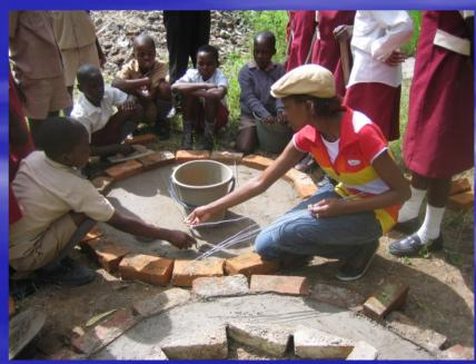
Once the concrete slab has been properly cured by leaving it covered and wet for a week before moving, it can be used to make a wide range of toilets.
