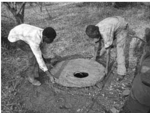
Figure 3-49: Slab placed over ring beam
