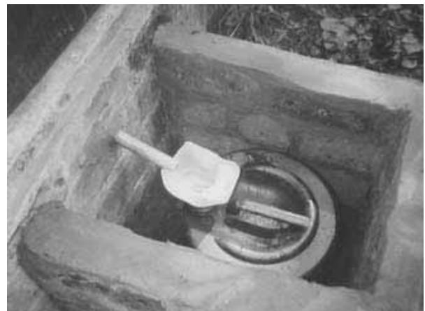
Figure 6-38: Plastic container that receives the urine from the urine-diverting toilet
