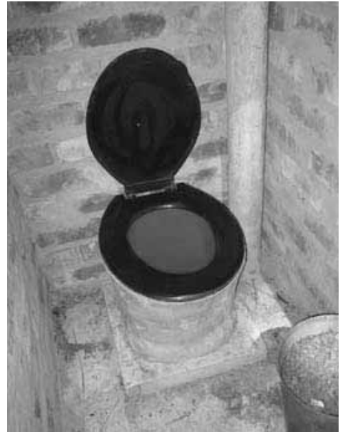
Figure 5-12: Completed low cost pedestal with plastic seat
