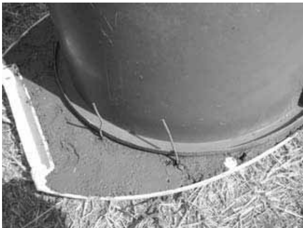
Figure 6-19: Bent wire added around the bucket
