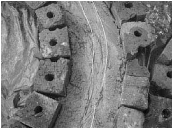
Figure 3-31: Wire reinforcement added
