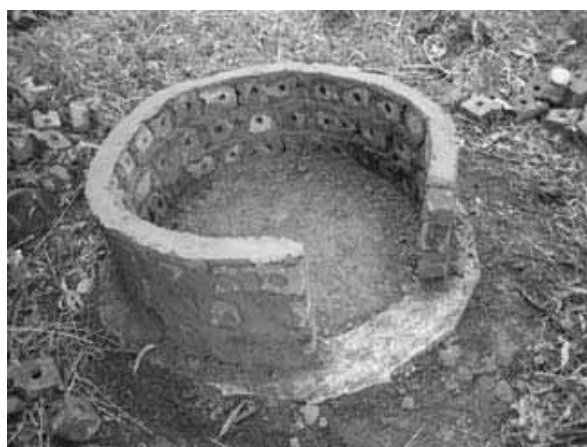
Figure 7-4: Brick wall built-up on ring beam
