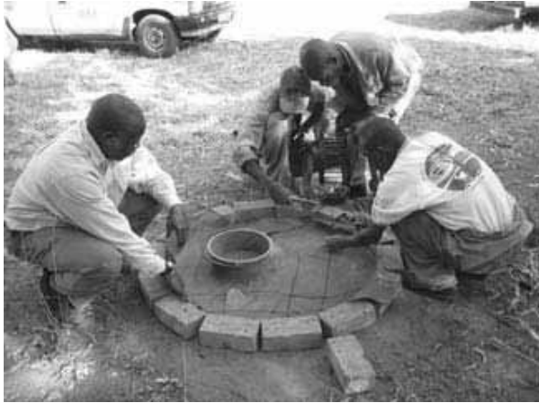
Figure 3-41: Laying down reinforcement wires
