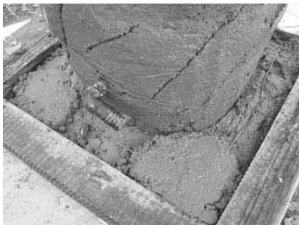
Figure 6-23: Wire added for reinforcement
