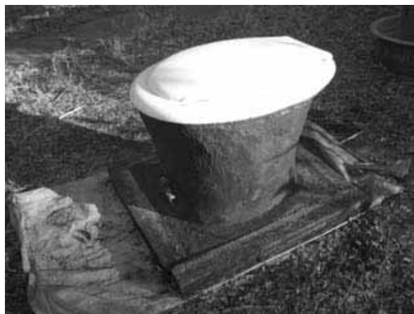
Figure 6-24: Completed pedestal curing
