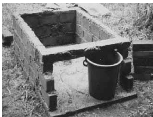
Figure 6-4: Testing the height of the vault access
