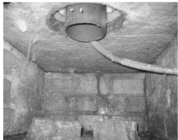
Figure 7-14: Urine pipe located below the slab
