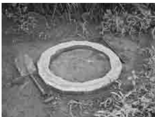
Figure 3-17: Completed ring beam
