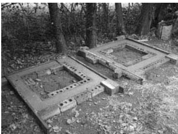
Figure 6-47: Casting ring beams
