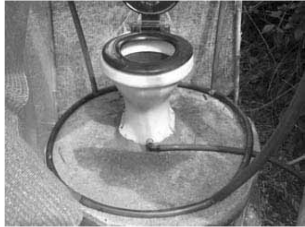
Figure 7-8: Urine-diverting pipe attached to base of pedestal
