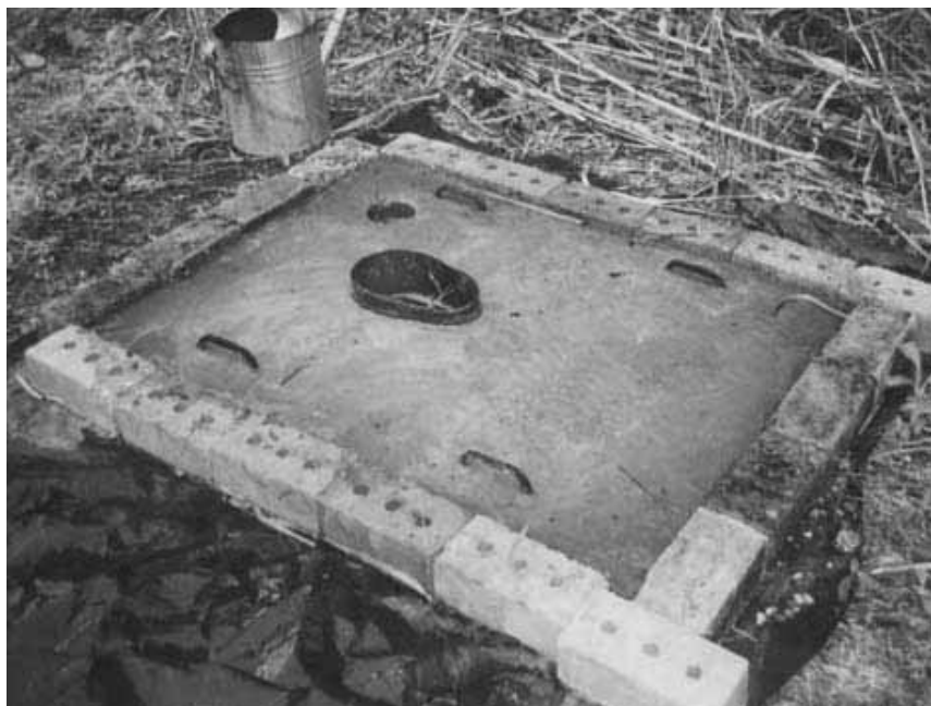
Figure 4-7: The completed slab inside the mould
