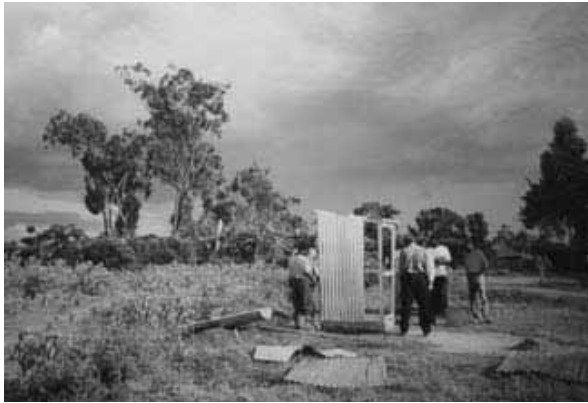
Figure 4-25: Construction of a portable structure for a Fossa alterna
