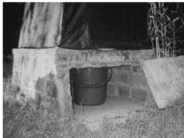
Figure 6-40: Internal view of vault with plastic bucket placed for collection of faeces
