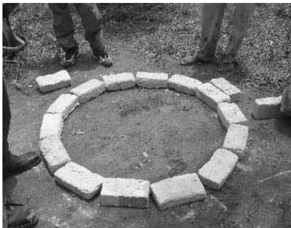
Figure 3-5: Ring of bricks for the mould
