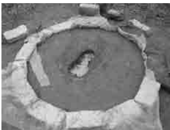
Figure 3-9: Mould after removal of squat hole insert
