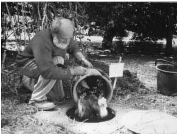
Figure 6-45: Emptying faeces into a small shallow pit
