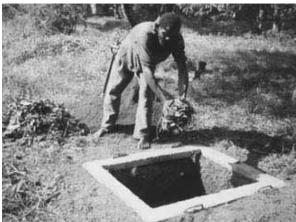
Figure 4-11: Adding leaves to the Fossa alterna pit
