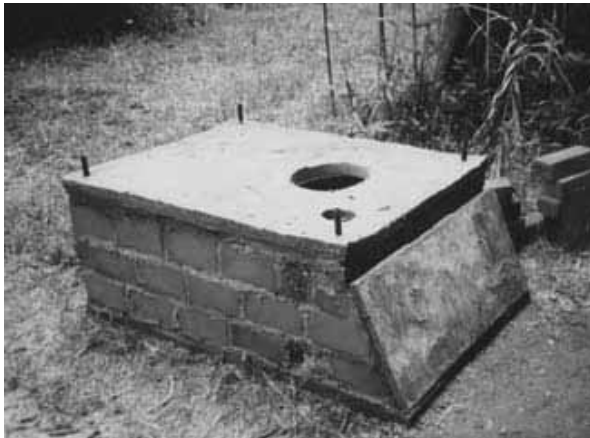
Figure 6-5: Fitting the vault access slab
