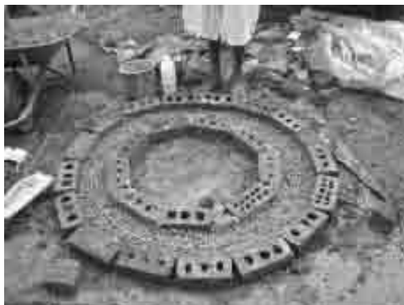
Figure 3-15: Cement and wire reinforcement added to mould
