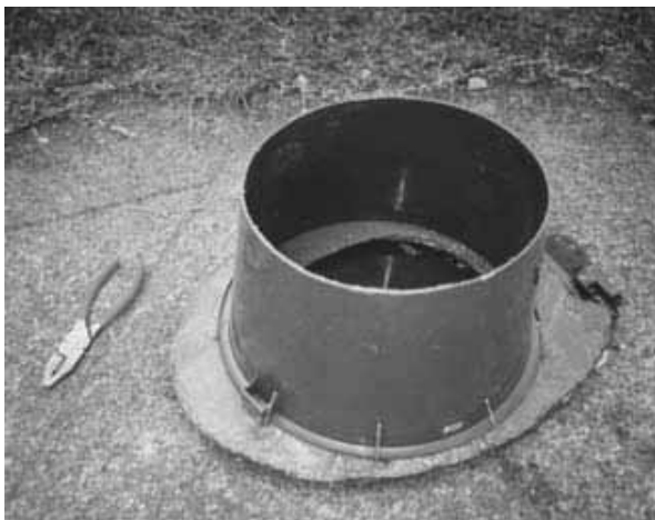
Figure 5-9: Plastic bucket placed over toilet seat
