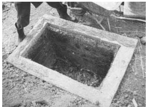
Figure 4-12: Completed Fossa alterna pit
