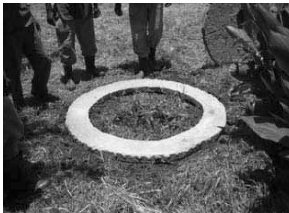
Figure 3-35: Placement of the concrete ring beam
