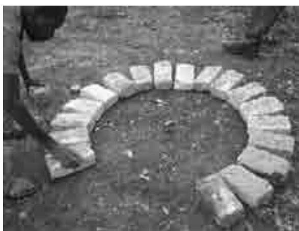
Figure 3-10: Forming the brick ring beam
