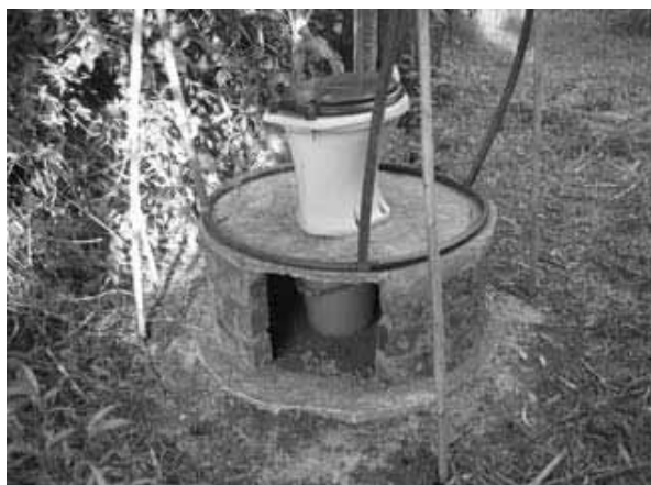
Figure 7-5: Slab and pedestal fitted on built-up base
