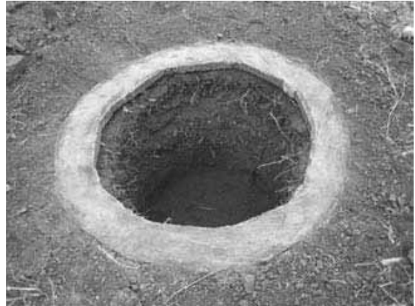
Figure 3-46: Pit dug inside ring beam
