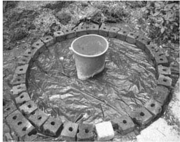
Figure 3-23: Shaped bucket to make the squat hole
