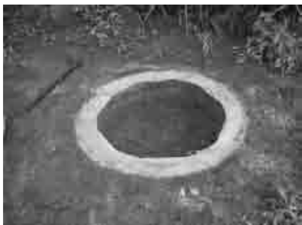
Figure 3-18: Digging of hole inside ring beam
