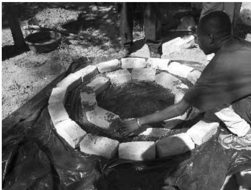
Figure 3-13: Brick mould on top of plastic sheet
