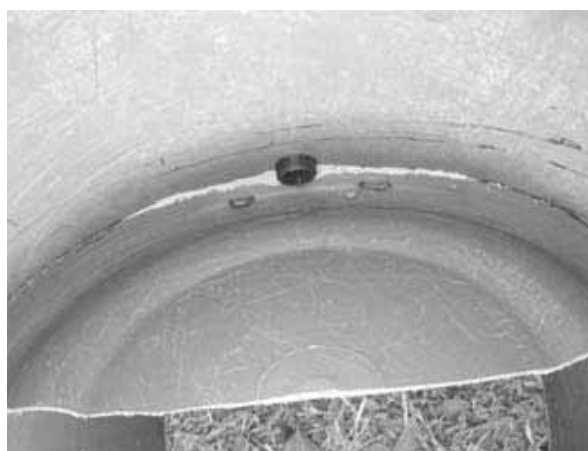
Figure 6-26: Sealing the top side of the urine diverter
