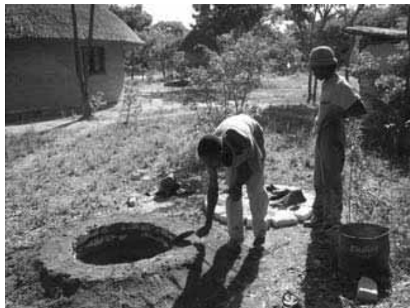
Figure 3-34: Packing soil around the brick ring beam
