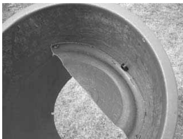
Figure 6-14: Inside view of the fitted pipe bend
