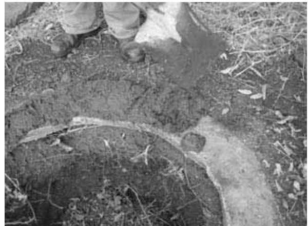
Figure 3-48: Anthill mortar packed around ring beam
