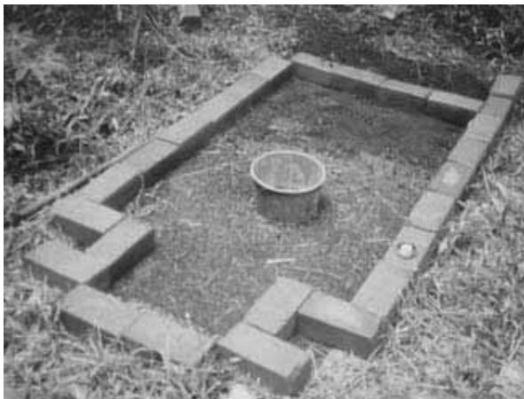
Figure 6-1: The brick mould for the base slab
