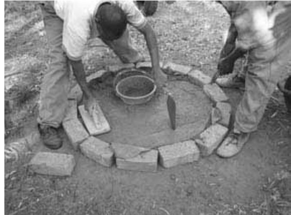
Figure 3-42: Levelling-off the concrete mix
