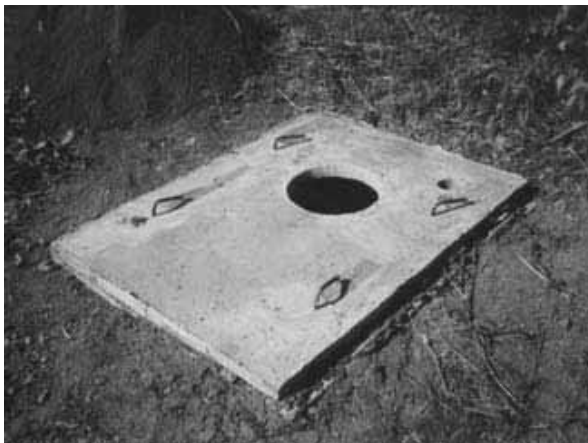
Figure 4-13: Addition of the concrete slab
