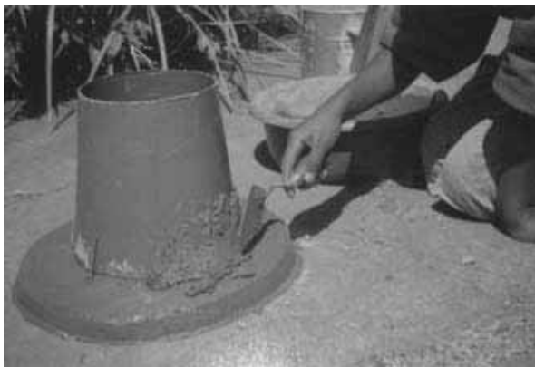
Figure 5-1: Construction of the very low cost pedestal
