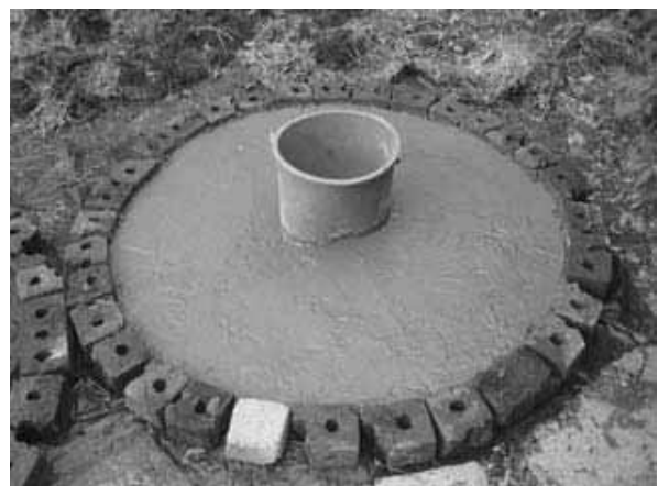
Figure 3-27: Remainder of concrete mix added and levelled-off
