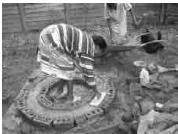
Figure 3-16: Levelling off the concrete
