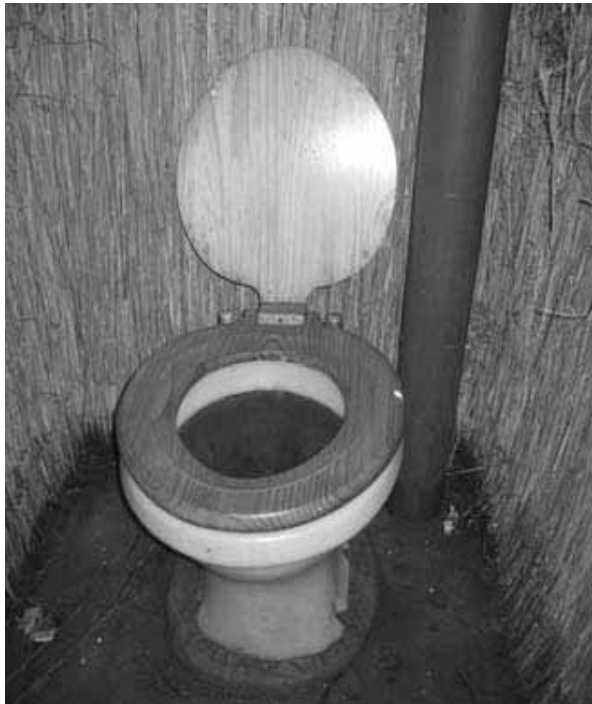
Figure 7-11: Fossa alterna upgraded with a non urine-diverting pedestal
