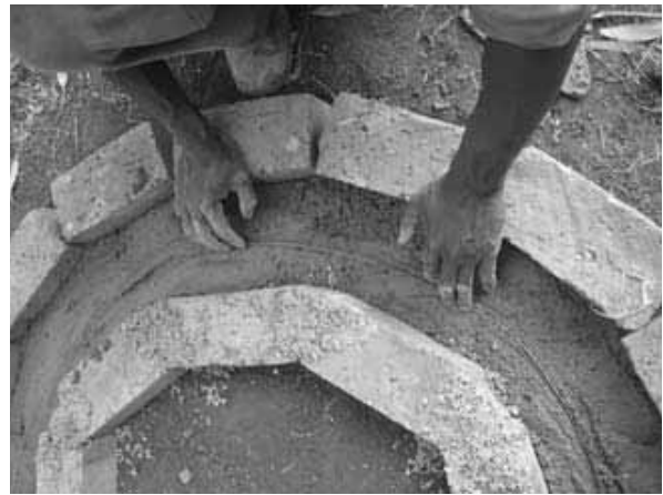
Figure 3-44: Addition of wire for reinforcement
