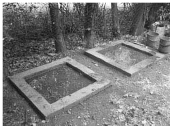
Figure 6-48: Cured ring beams
