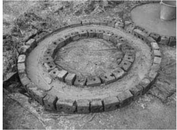
Figure 3-30: Concrete mix added to mould
