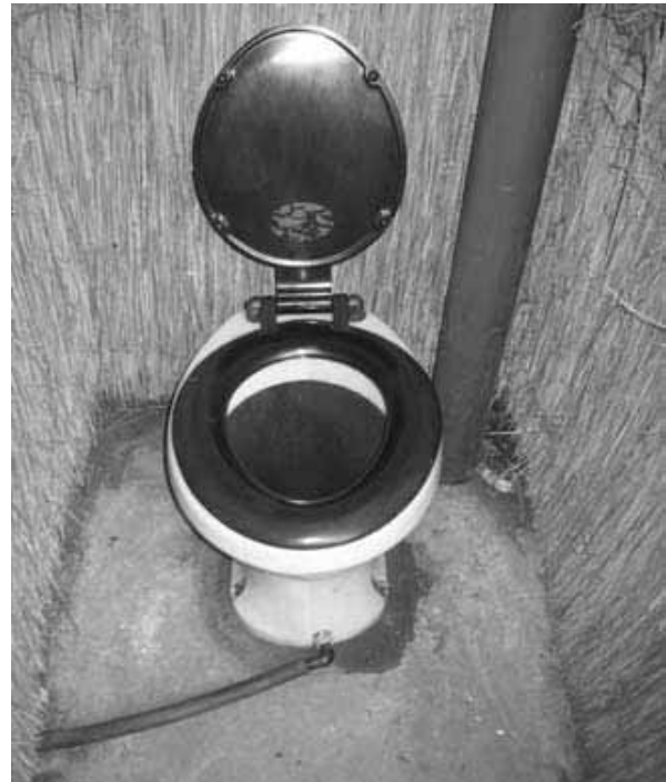
Figure 7-12: Fossa alterna upgraded with a urine-diverting pedestal
