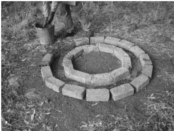
Figure 3-43: Ring beam mould using bricks
