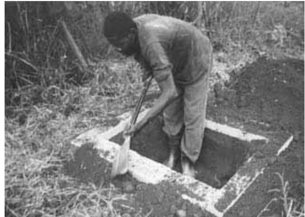
Figure 4-10: Digging the pit for the Fossa alterna
