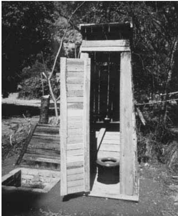
Figure 4-15: Fossa alterna using a wooden structure
