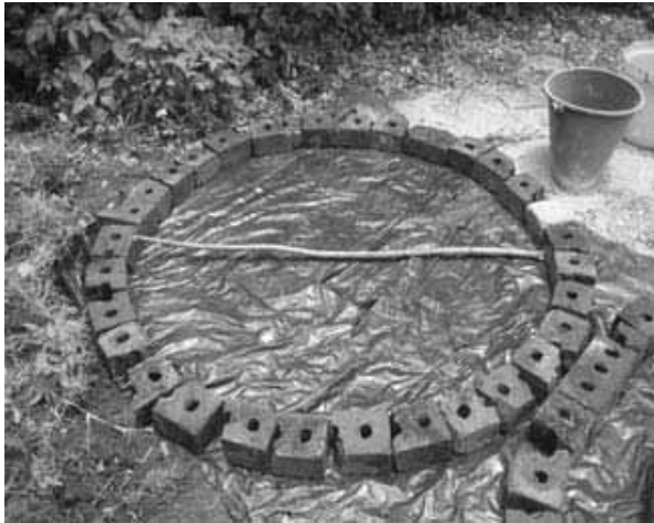
Figure 3-22: Circle of bricks 1.15m in diameter
