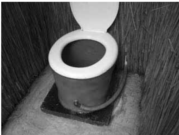
Figure 6-31: Urine-diverting pedestal installed
