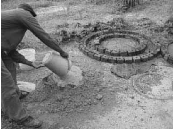
Figure 3-29: Mixing the cement and river sand
