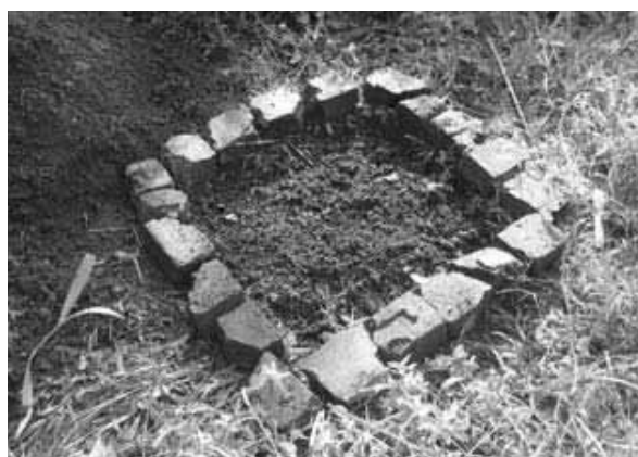
Figure 10-16: Bricks laid around the tree pit
