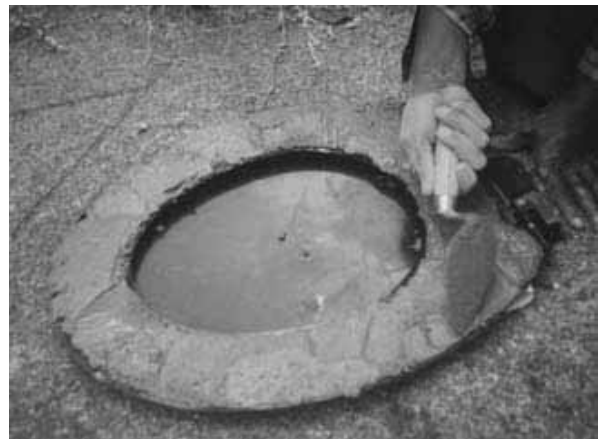
Figure 5-8: Plastic toilet seat filled with strong concrete
