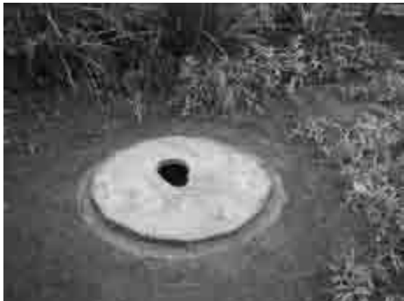
Figure 3-20: Toilet slab placed on ring beam
