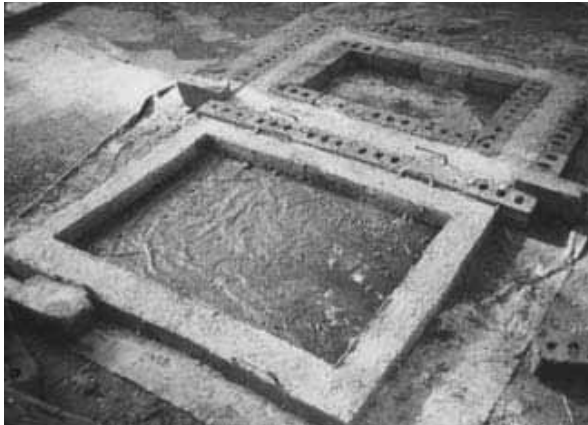
Figure 4-9: Ring beam mould using bricks
