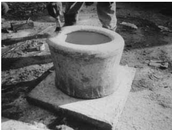
Figure 5-5: Painting the concrete pedestal
