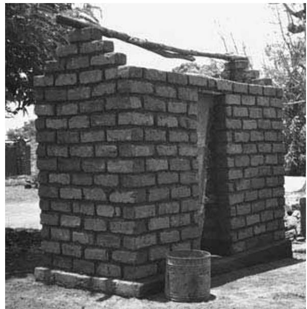
Figure 4-28: Brick double pit composting toilet
