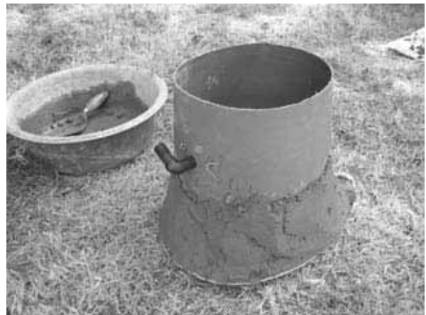
Figure 6-20: Concrete added half-way up the bucket
