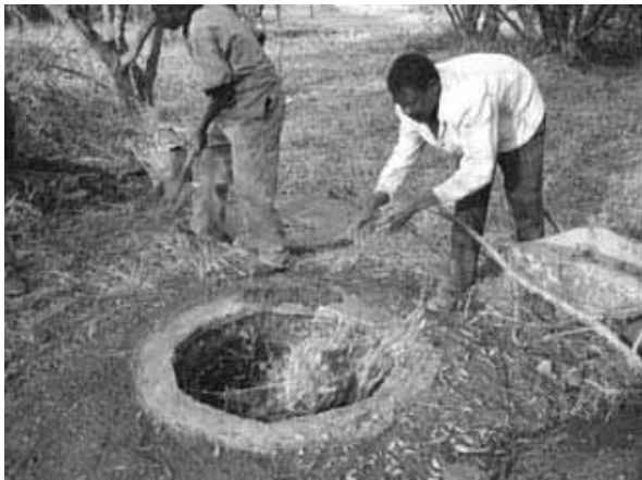
Figure 3-47: Addition of leaves to pit
