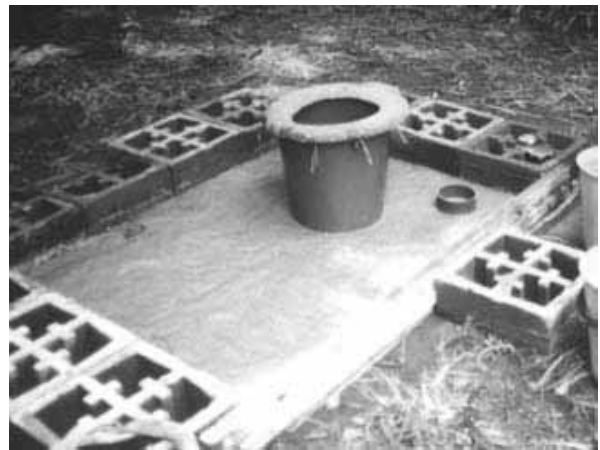
Figure 6-2: The brick mould for the toilet slab
