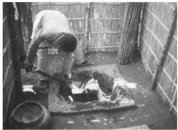
Figure 4-22: Excavating the humus from the pit
