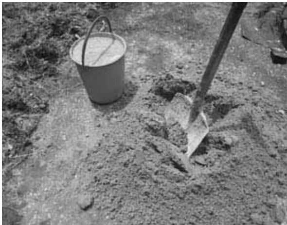
Figure 3-24: Mixing the cement and river sand
