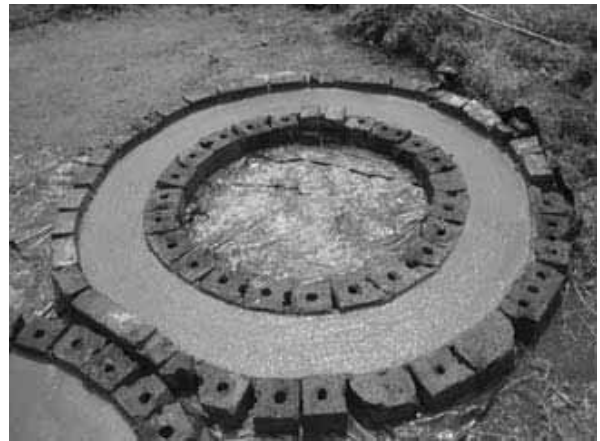
Figure 3-32: Remainder of concrete mix added and levelled-off
