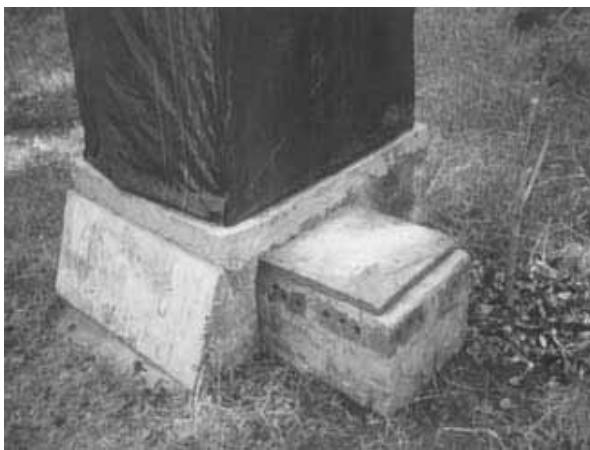
Figure 6-39: Side-vault for urine collection
