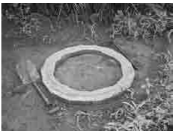
Figure 7-3: Ring beam laid on level ground
