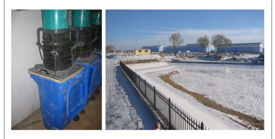
(left) Bins in basement containing dry faeces mixed with dry cellulose fibre – drying & bulking agent & carbon source for later composting
