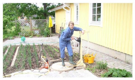
Figure 20. Hand pumping of urine from household tank for subsequent use in garden. Photo: Mats Johansson.
