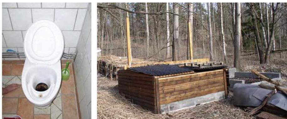
Figure 14. (left) The sanitation system is unique: a urine-diverting system with dry collection of faeces in a 2-storey building. Photo: Mats Johansson.
